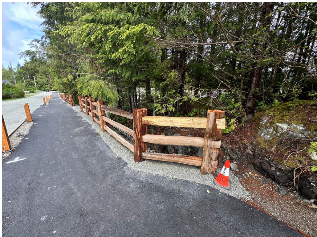
Photo #6 – Split Rail Fencing Installation
