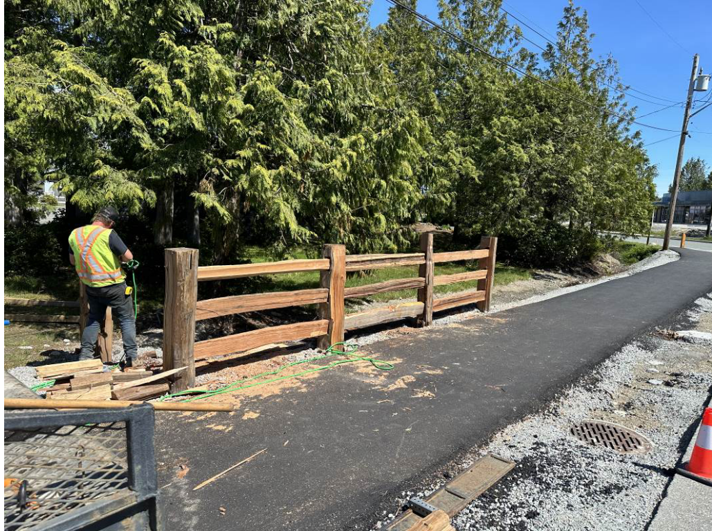
Photo #3 – Split Rail Fencing Installation
