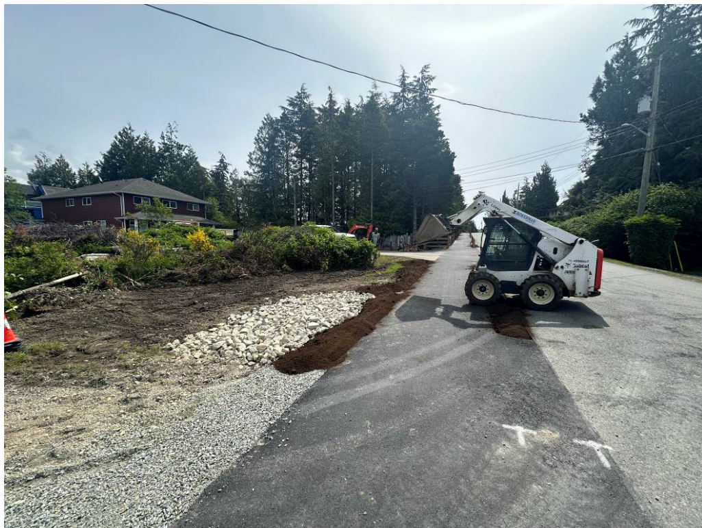
Photo #8 – Growing Medium Placement & Rock Pit Installation
