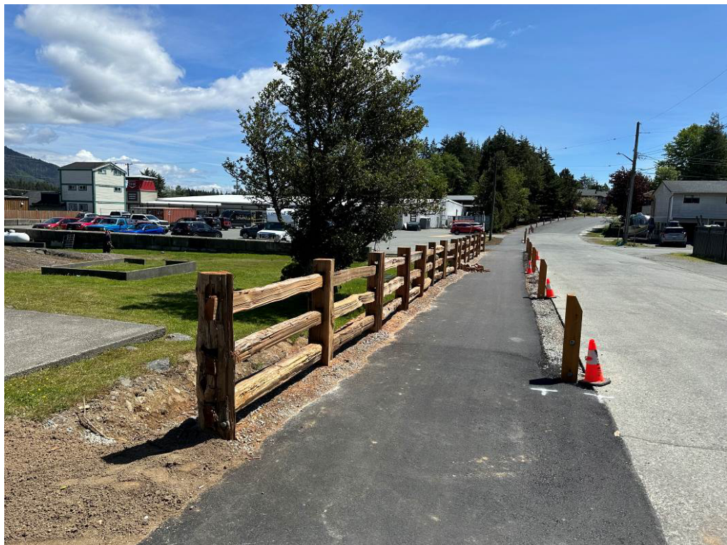
Photo #4 – Split Rail Fencing Installation
