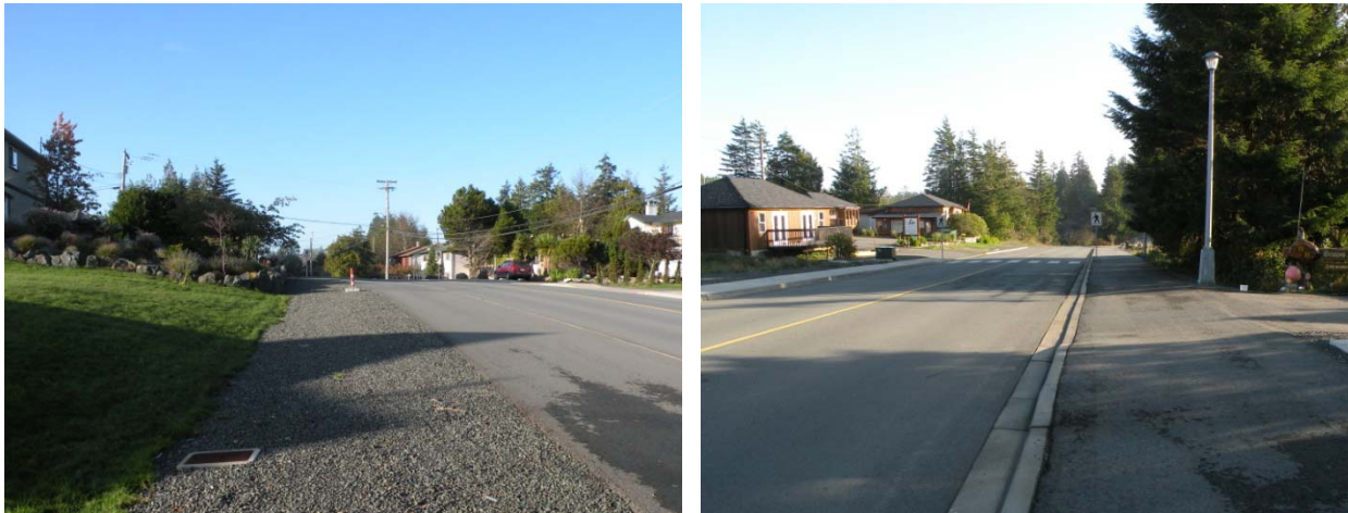
Figure 15: New road sections on Peninsula Road, between Little Beach and Marine Drive.
