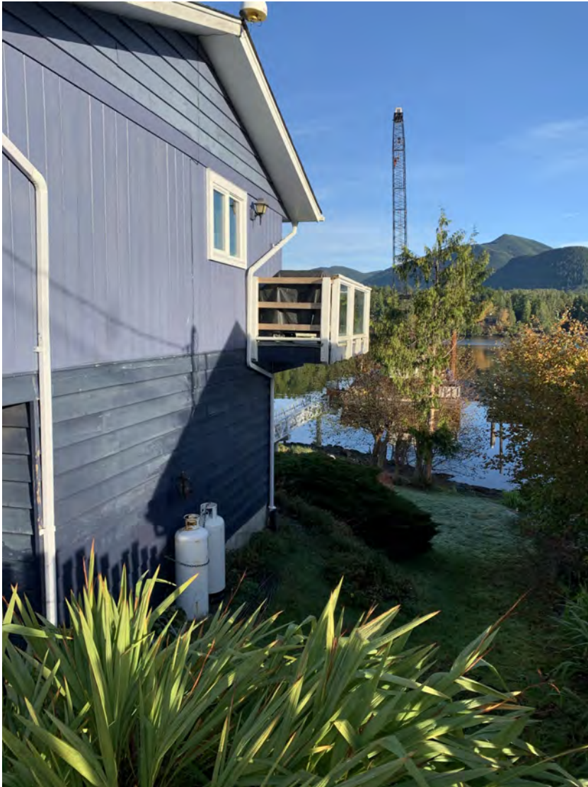
Photo 3. Photo of 1567 Imperial Lane showing the east side of the residence. (November 16, 2023)
