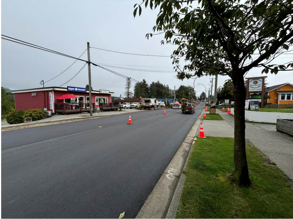
Photo #7 – Asphalt Paving (Base Lift)
