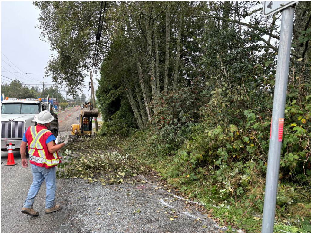
Photo #4 – Clearing / Trimming for Roadway Widening
