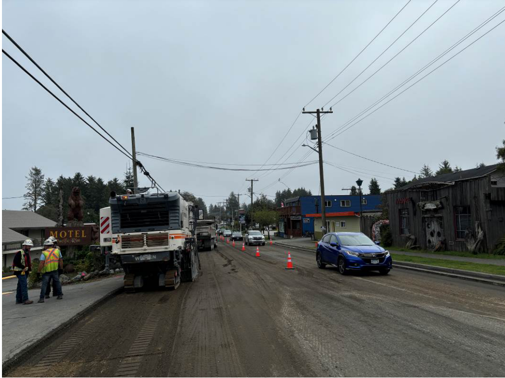
Photo #1 – Asphalt Removal (Milling)
