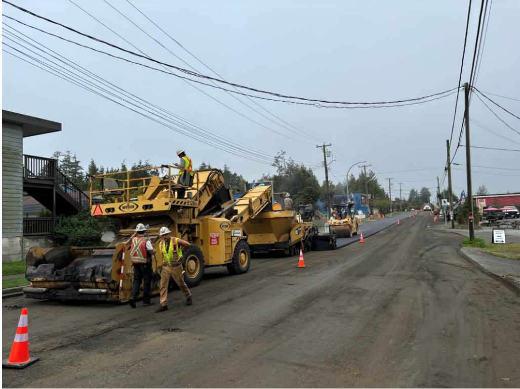
Photo #5 – Asphalt Paving (Base Lift)
