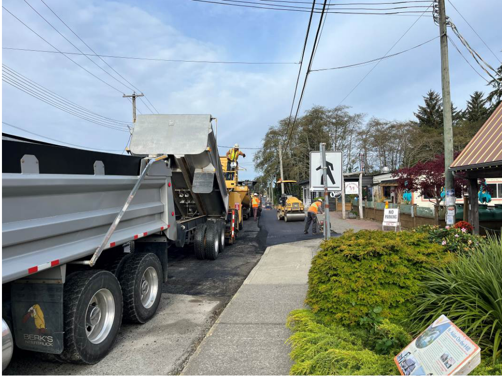
Photo #13 – Asphalt Paving (Top Lift)
