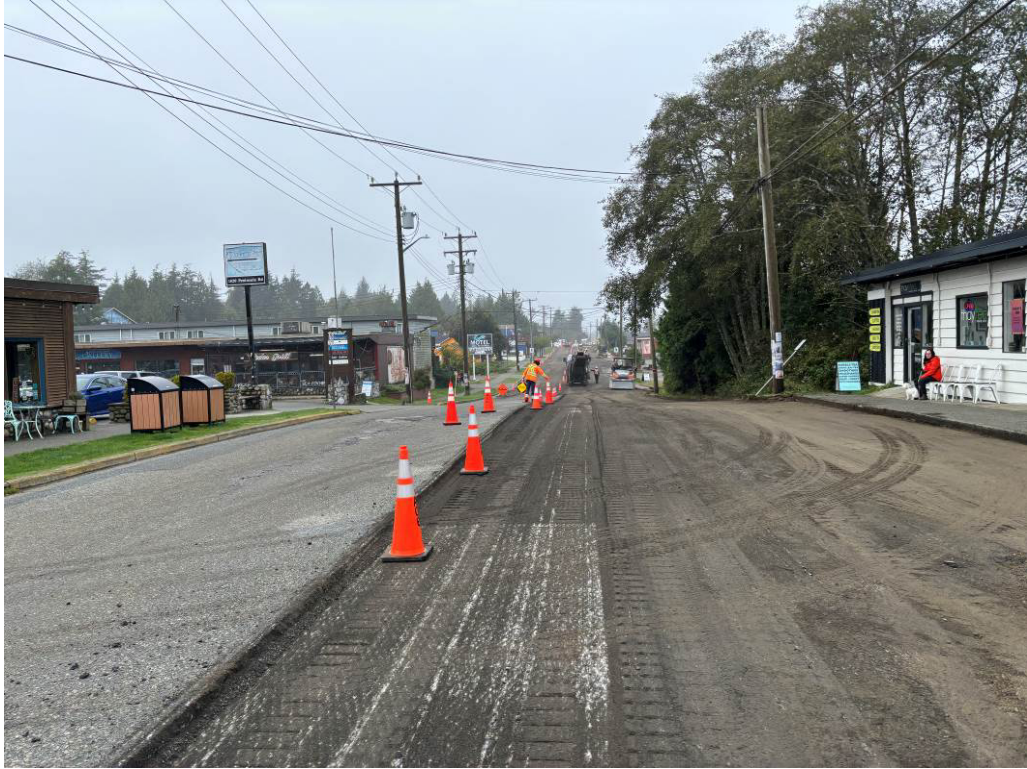
Photo #3 – Asphalt Removal (Milling)
