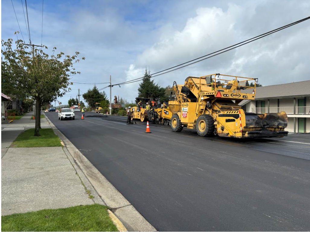
Photo #11 – Asphalt Paving (Top Lift)
