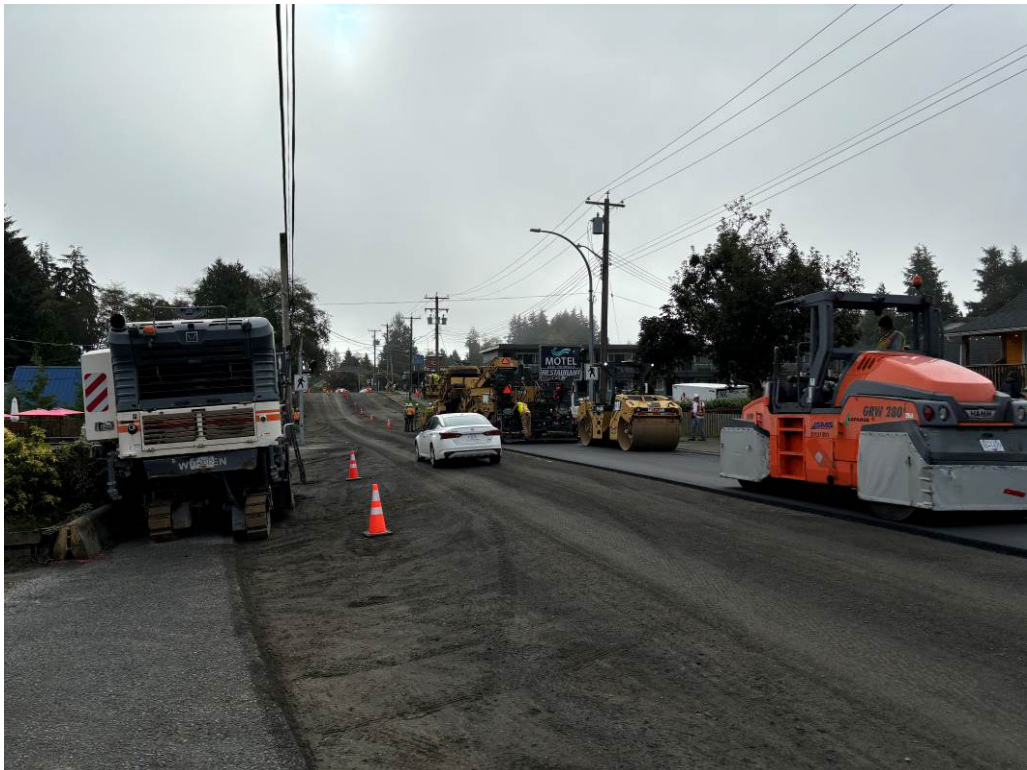
Photo #6 – Asphalt Paving (Base Lift)
