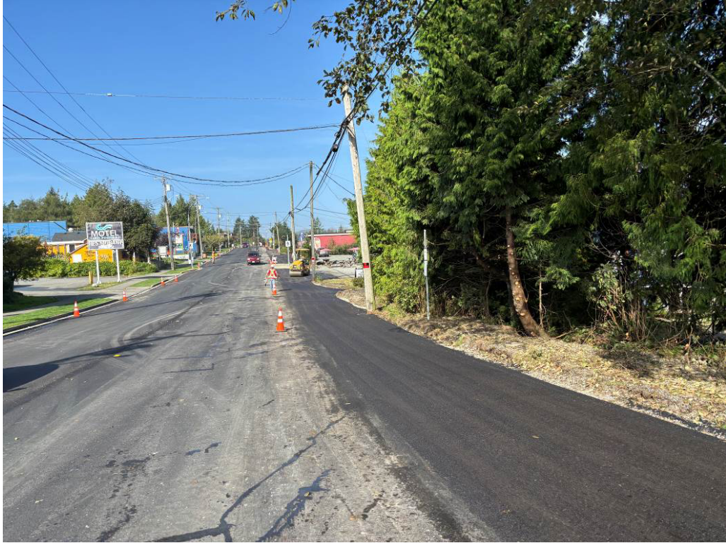
Photo #9 – Asphalt Paving (Base Lift)
