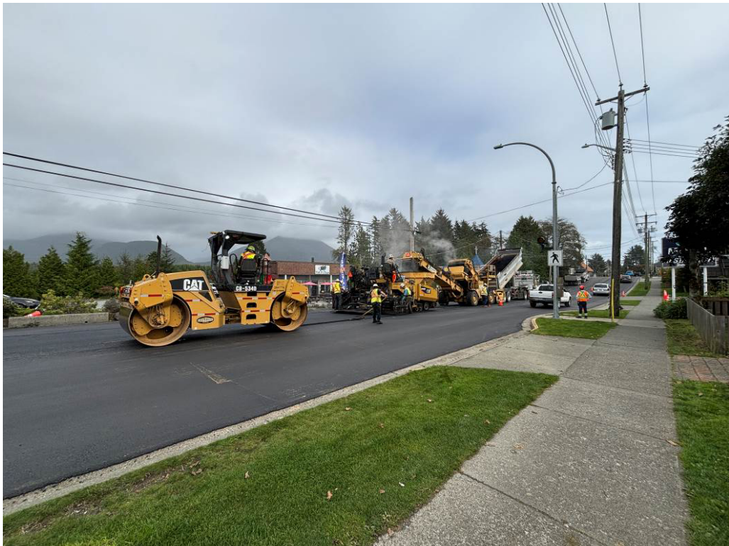
Photo #13 – Asphalt Paving (Top Lift)
