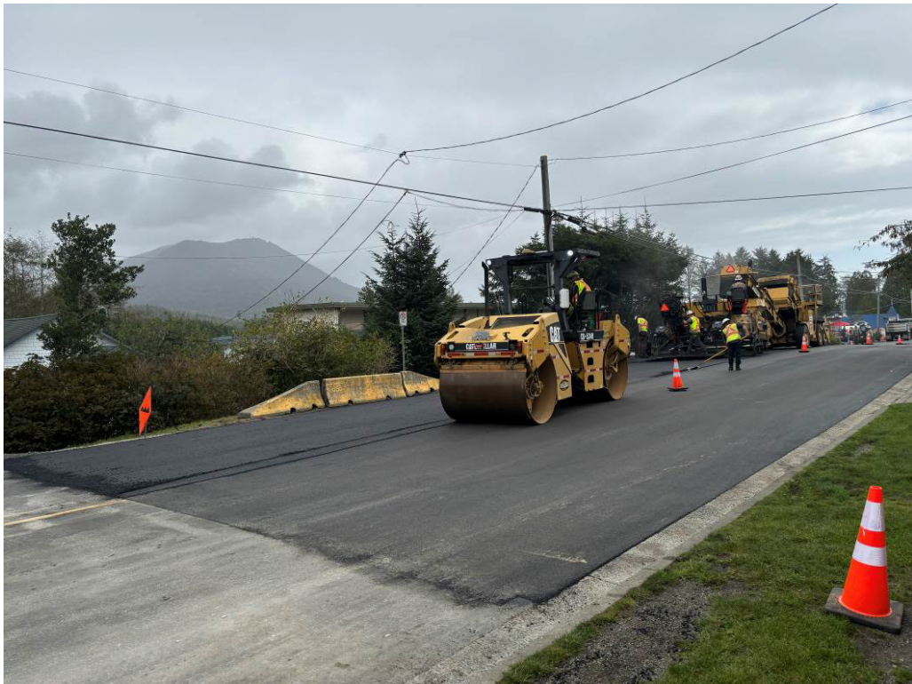
Photo #10 – Asphalt Paving (Top Lift)
