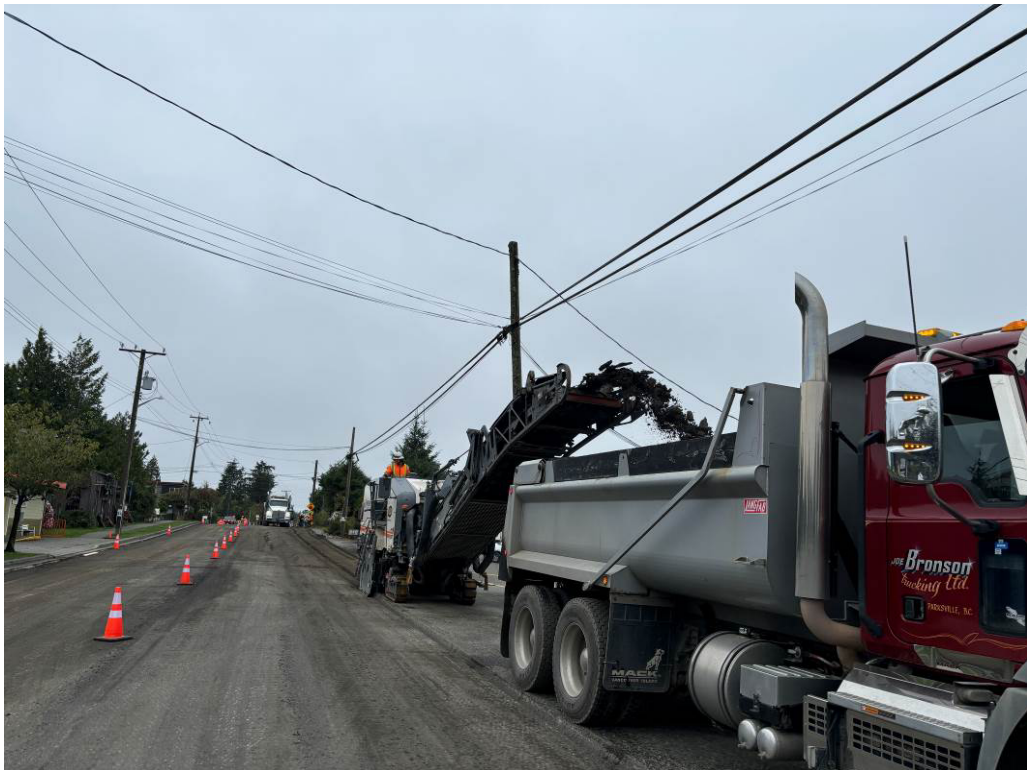
Photo #2 – Asphalt Removal (Milling)
