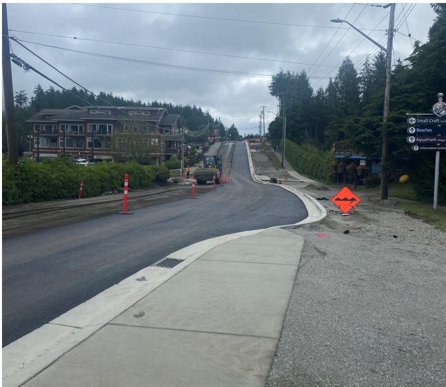
Photo #6 – Roadway Paving (Bottom Lift) Ongoing
