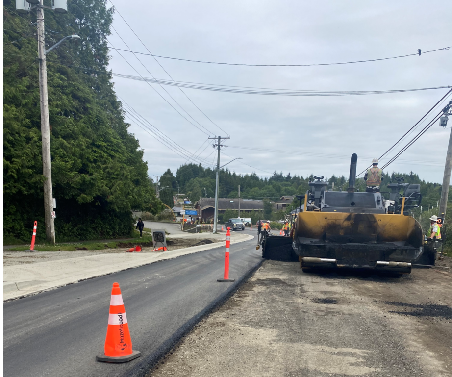
Photo #5 – Roadway Paving (Bottom Lift) Ongoing
