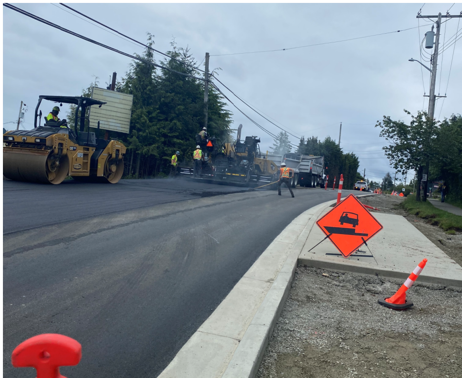
Photo #4 – Roadway Paving (Bottom Lift) Ongoing
