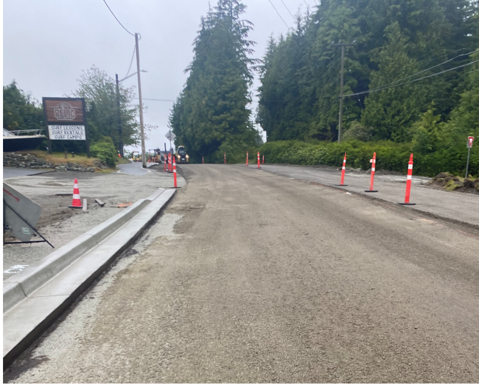
Photo #1 – Roadway Grading Ongoing
