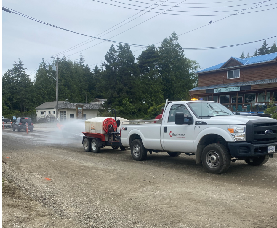
Photo #3 – Dust Control Ongoing
