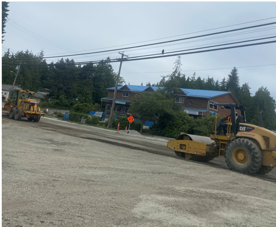
Photo #2 – Roadway Widening Ongoing
