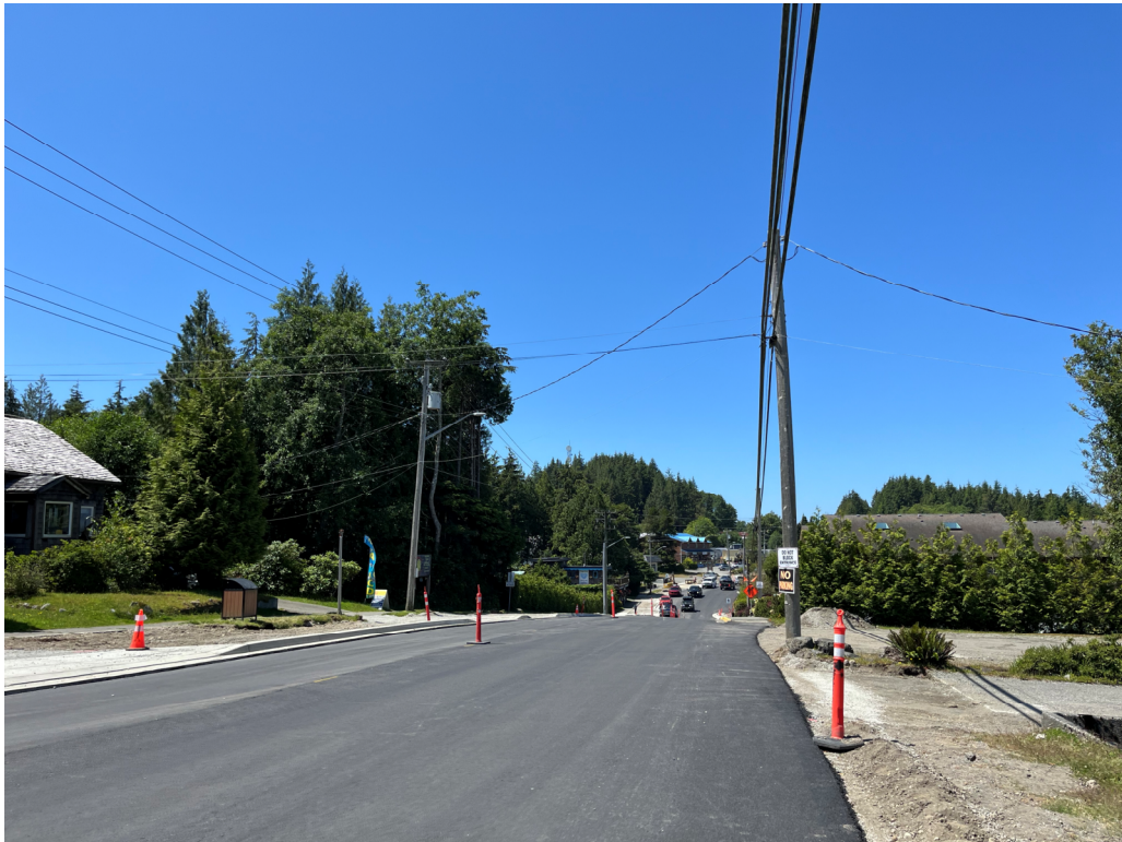
Photo #8 – Roadway Paving (Bottom Lift) Ongoing
