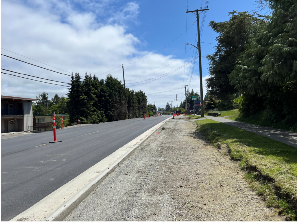
Photo #7 – Roadway Paving (Bottom Lift) Ongoing
