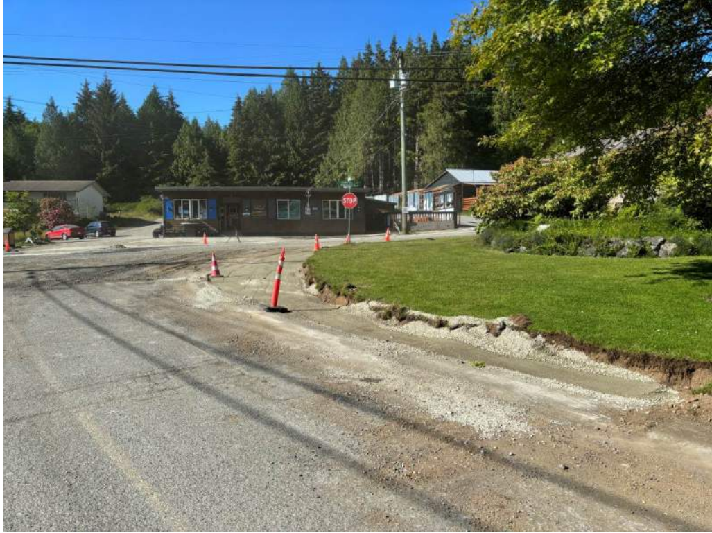
Photo #3 – Roadway Widening Ongoing
