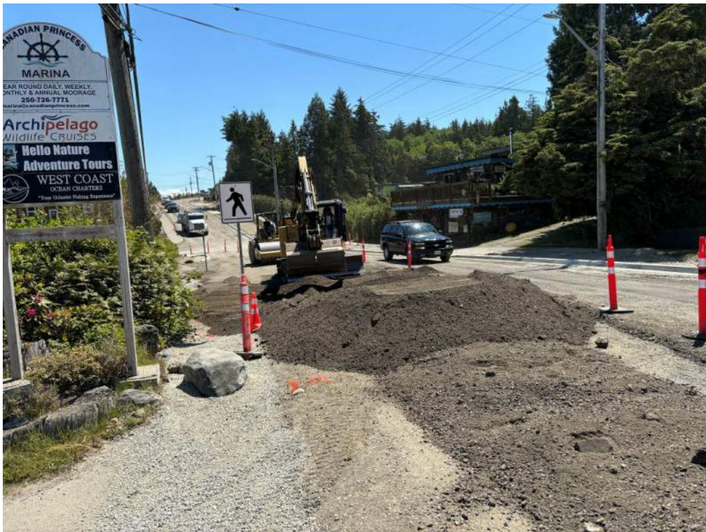
Photo #2 – Roadway Widening Ongoing
