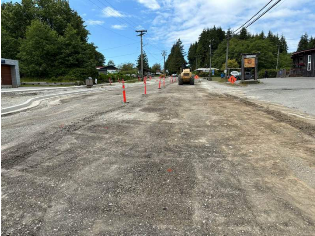
Photo #1 – Roadway Grading Ongoing
