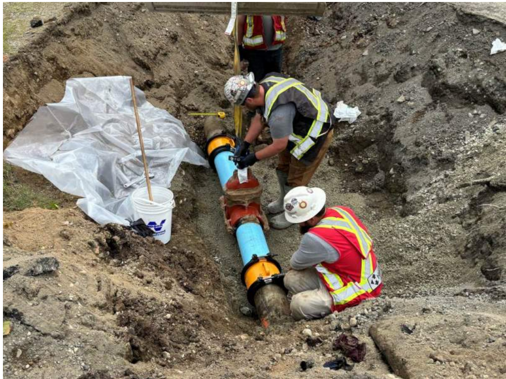
Photo #6 – Failed Water Valve Replaced (1 of 3)
