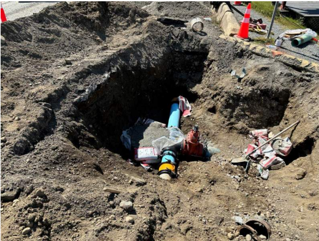
Photo #8 – Failed Water Valve Replaced (3 of 3)
