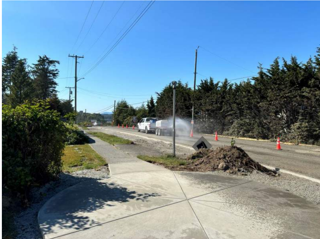
Photo #5 – Dust Control Ongoing
