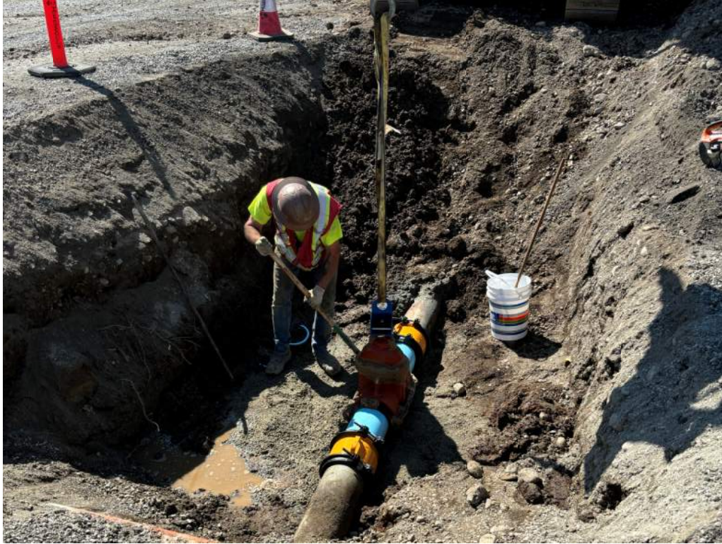
Photo #7 – Failed Water Valve Replaced (2 of 3)
