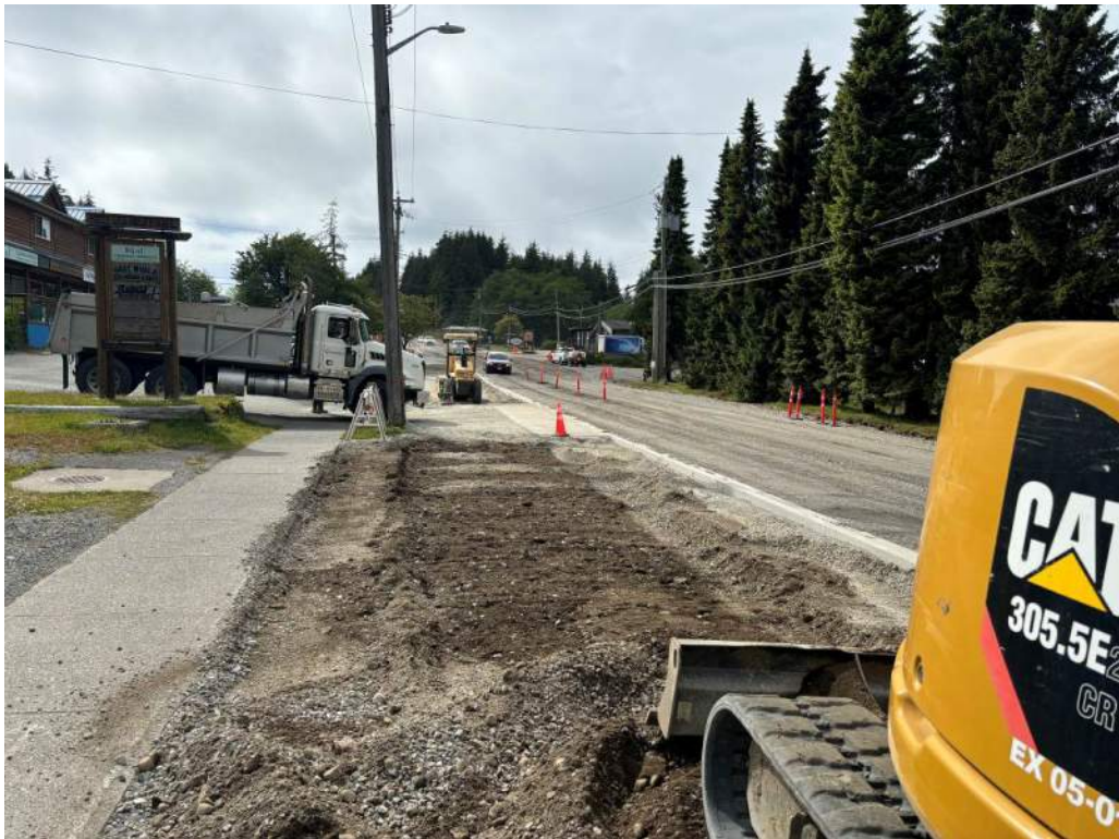
Photo #4 – Bike Track Grading Ongoing
