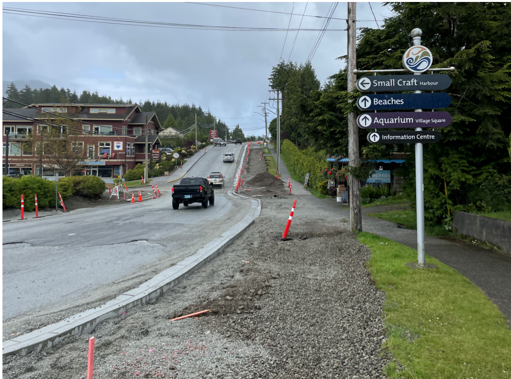
Photo #2 – Peninsula Road Curb Installation
