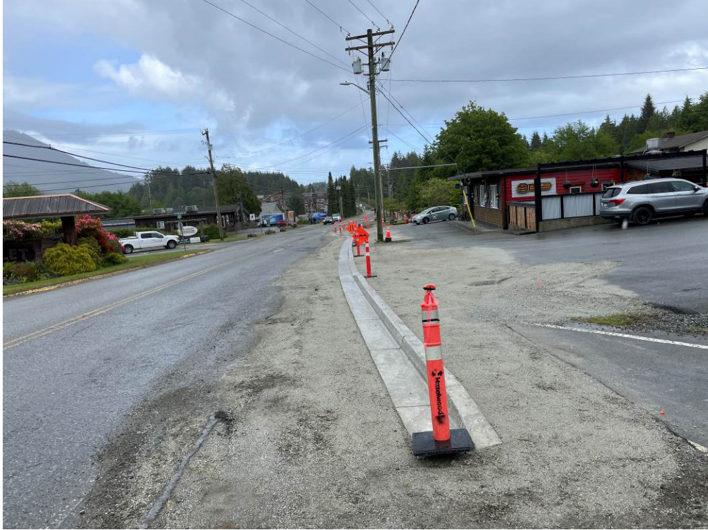
Photo #1 – Peninsula Road Curb Installation
