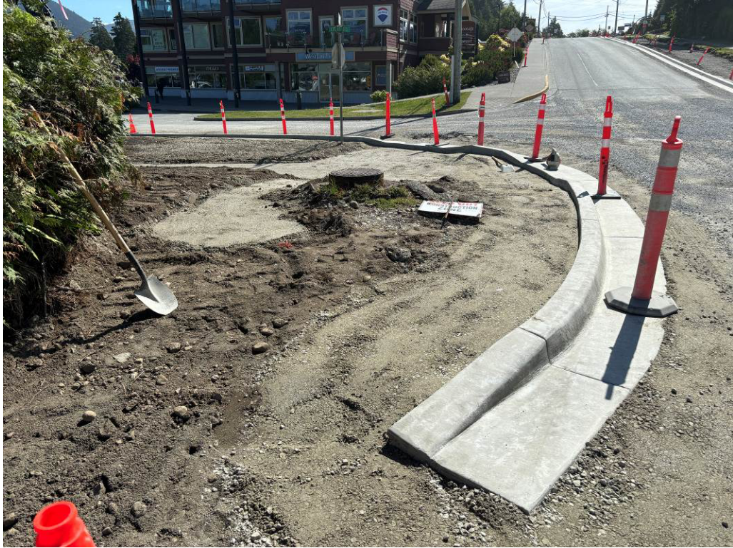
Photo #3 – Peninsula Road Curb Installation
