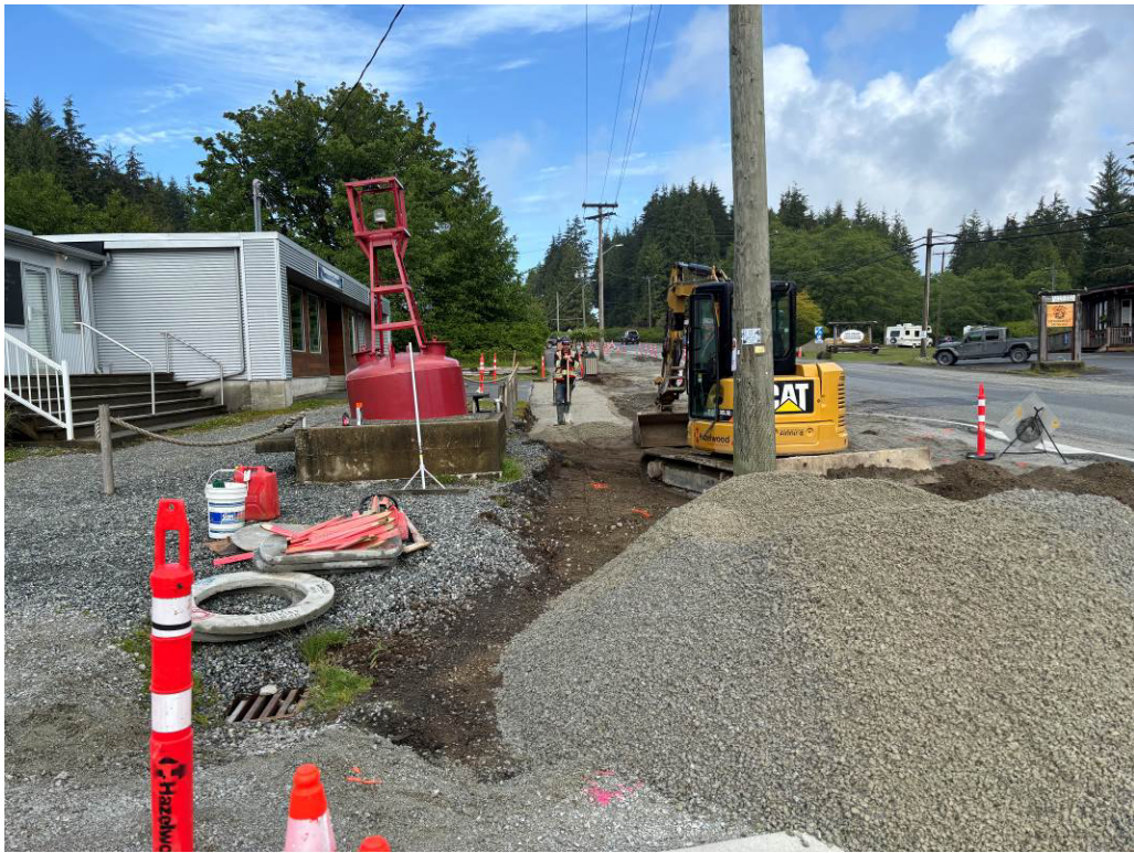
Photo #4 – Peninsula Road Boulevard / Sidewalk Prep
