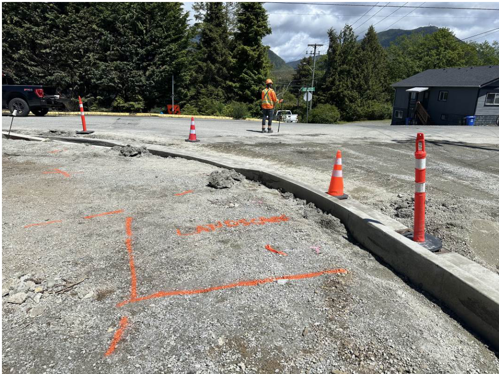
Photo #8 – Peninsula Road Concrete Works Layout Ongoing
