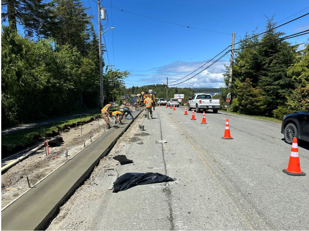
Photo #1 – Peninsula Road Curb Installation
