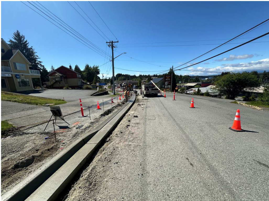
Photo #2 – Peninsula Road Curb Installation
