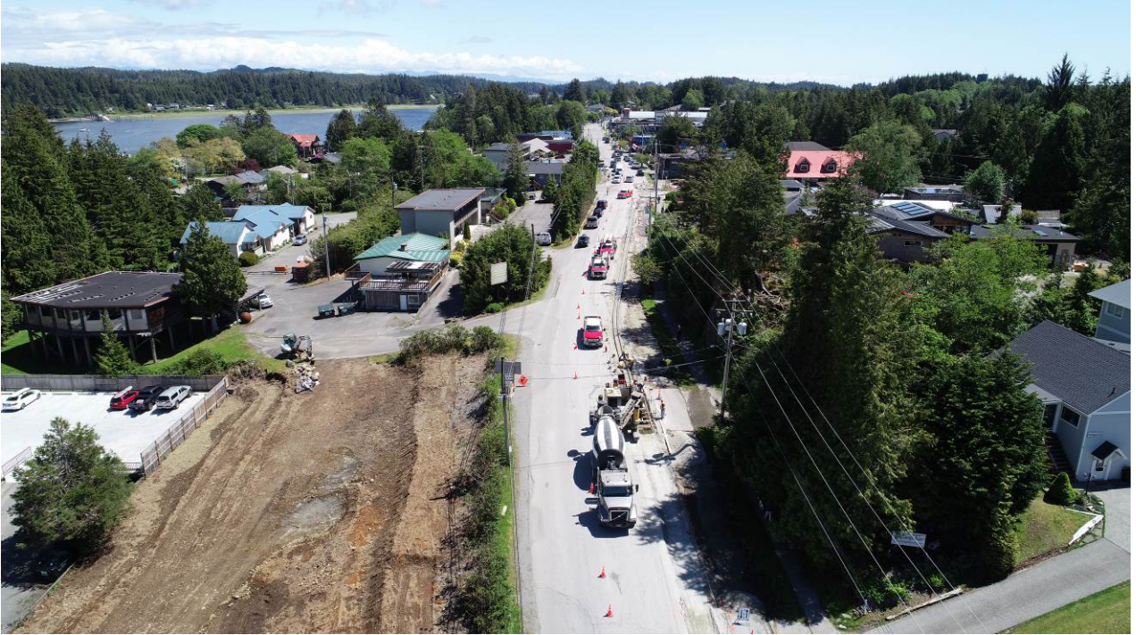
Photo #3 – Peninsula Road Curb Installation
