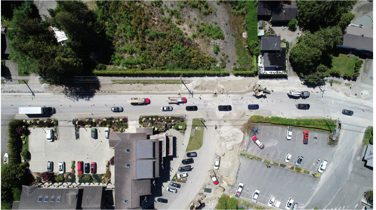
Photo #5 – Peninsula Road Curb Installation
