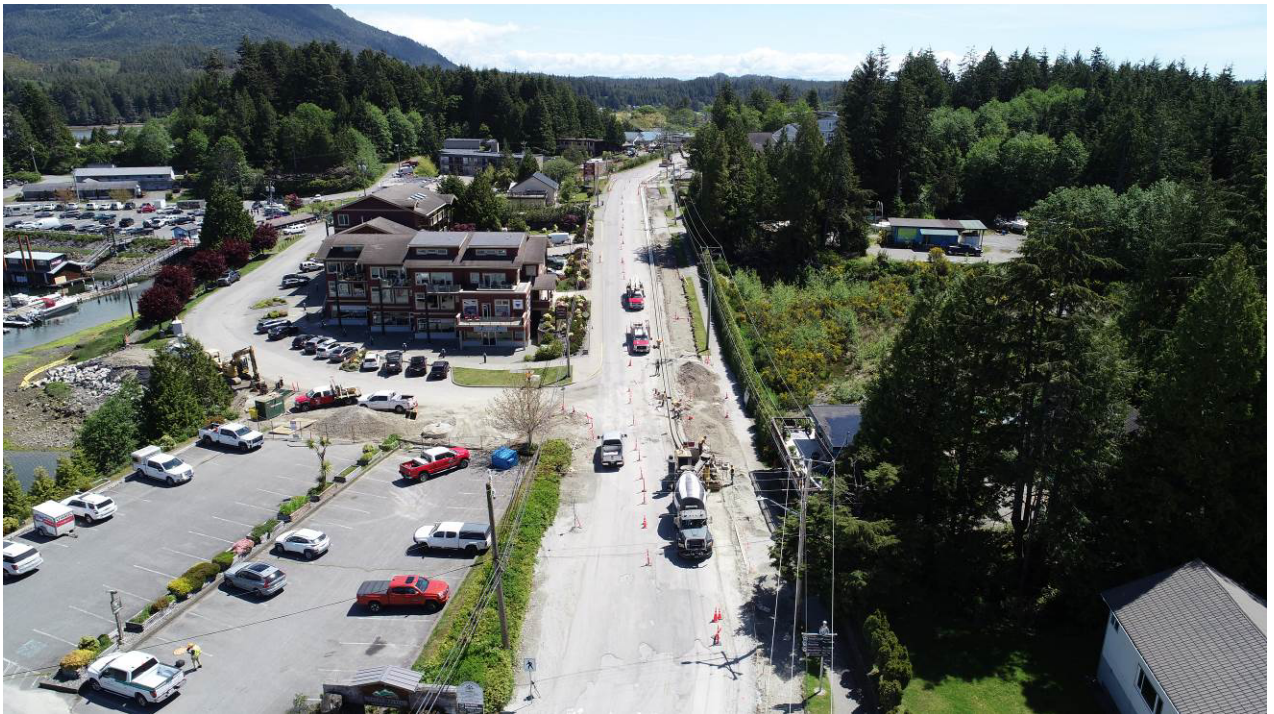
Photo #6 – Peninsula Road Curb Installation
