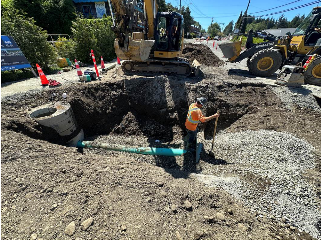
Photo #5 – Peninsula Road Sanitary Replacement (Lyche Rd Crossing)
