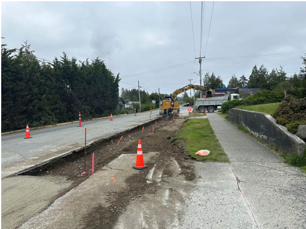
Photo #6 – Curb & Boulevard Preparation (Bay St) – Ongoing
