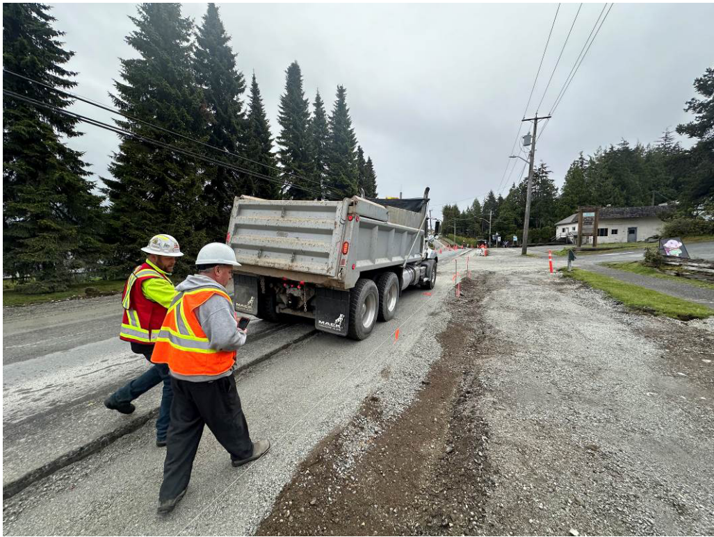
Photo #8 – Curb Base Proof Roll Test Completed
