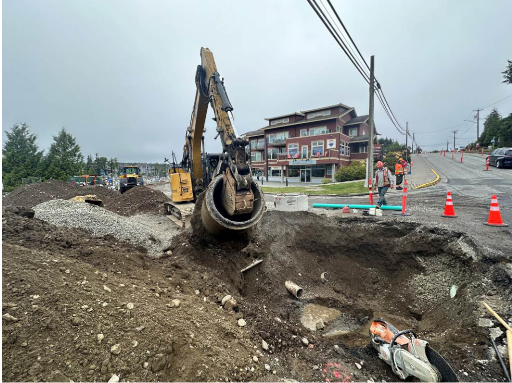
Photo #3 – Peninsula Road Sanitary Replacement (Lyche Rd Crossing – North MH Removal)
