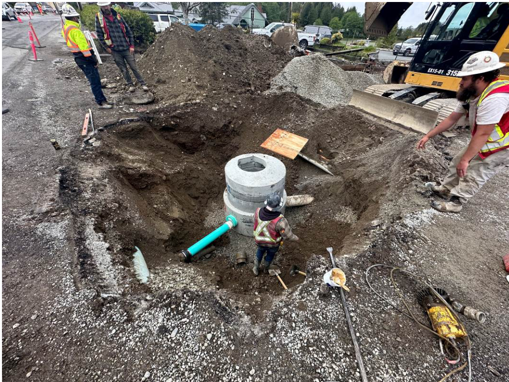
Photo #4 – Peninsula Road Sanitary Replacement (Lyche Rd Crossing – North MH)
