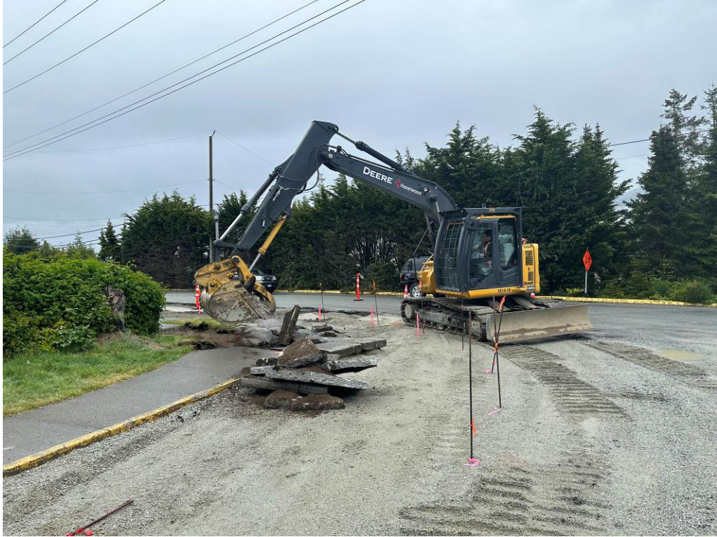
Photo #7 – Curb & Boulevard Preparation (Bay St) – Ongoing
