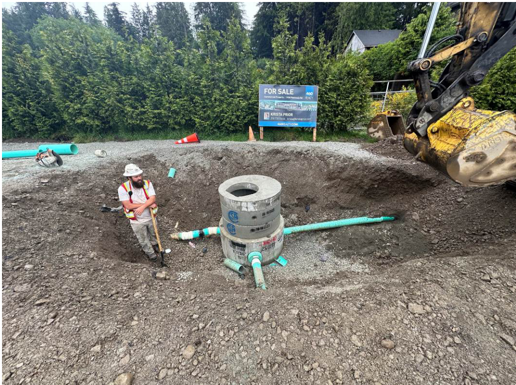
Photo #2 – Peninsula Road Sanitary Replacement (Lyche Rd Crossing – South MH)
