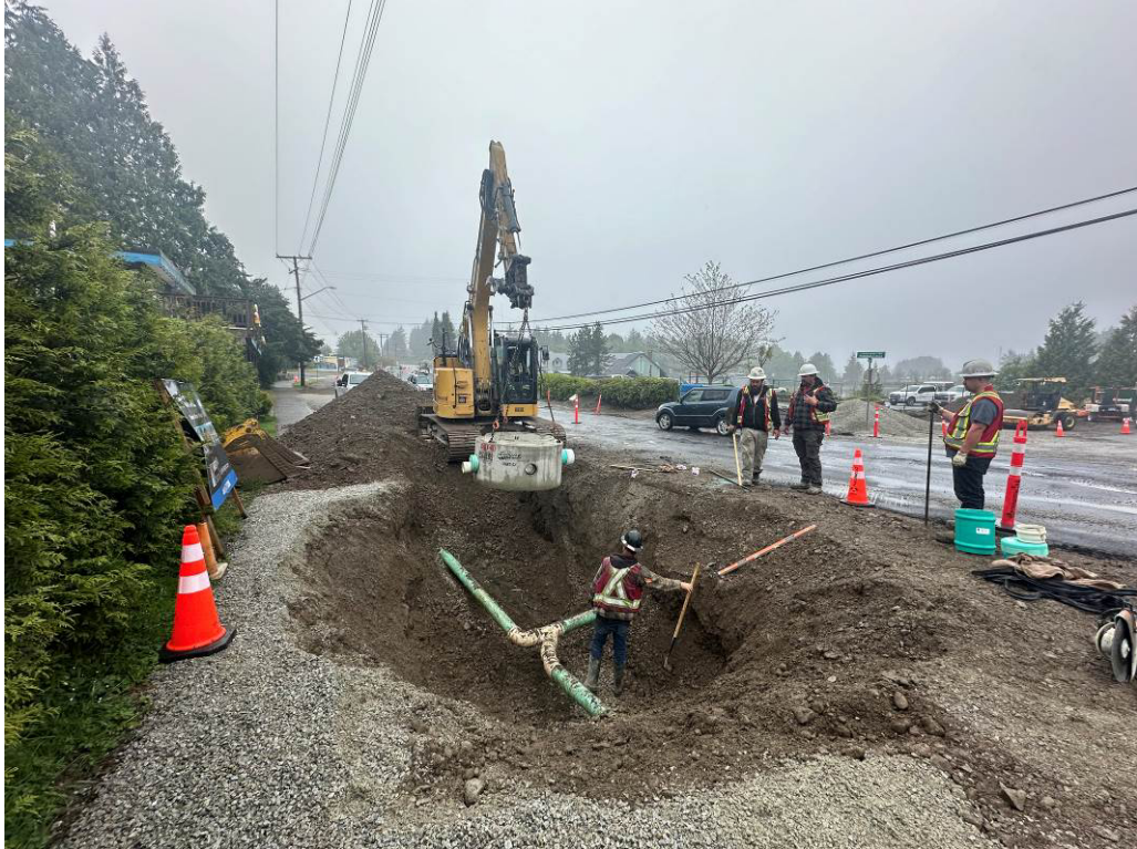
Photo #1 – Peninsula Road Sanitary Replacement (Lyche Rd Crossing – South MH)
