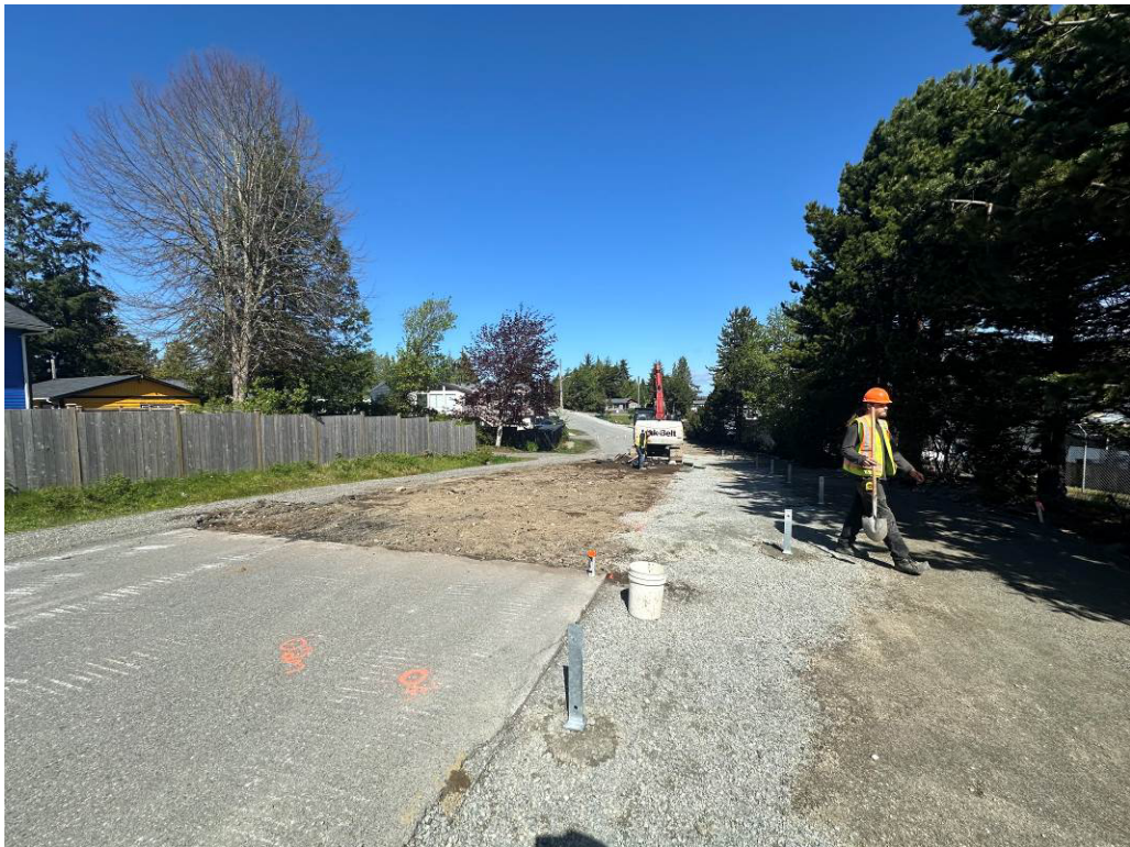
Photo #2 – Expanded Asphalt Removal & Replacement Preparation Completed
