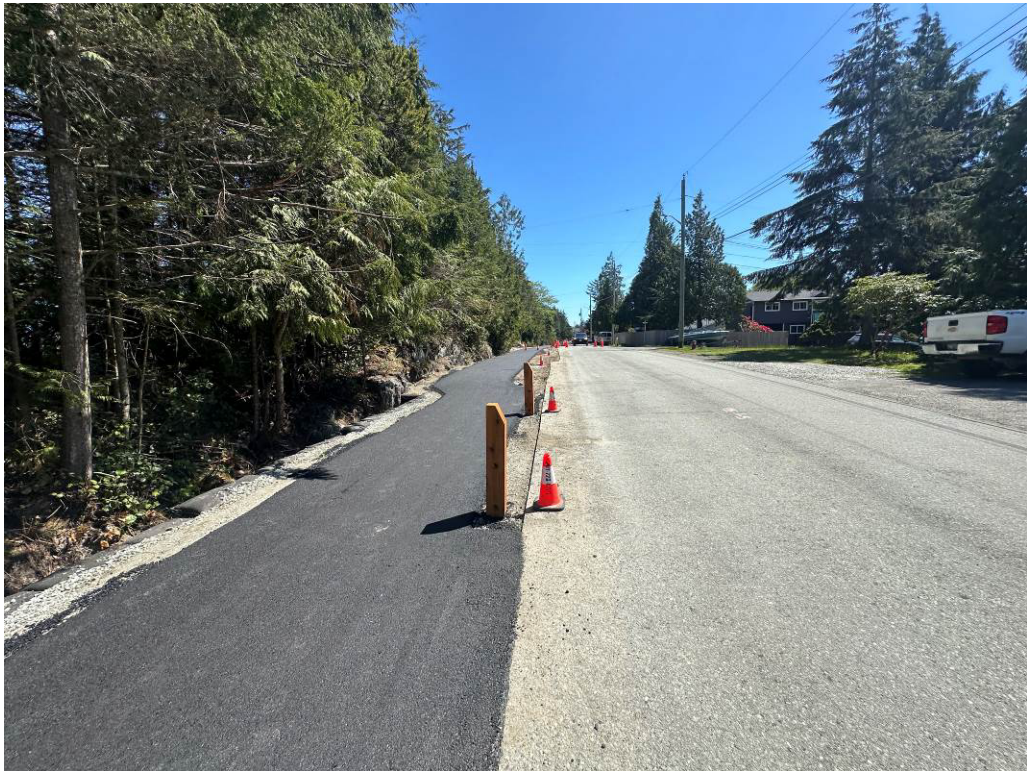
Photo #6 – Larch Road Pathway – Paving in Progress
