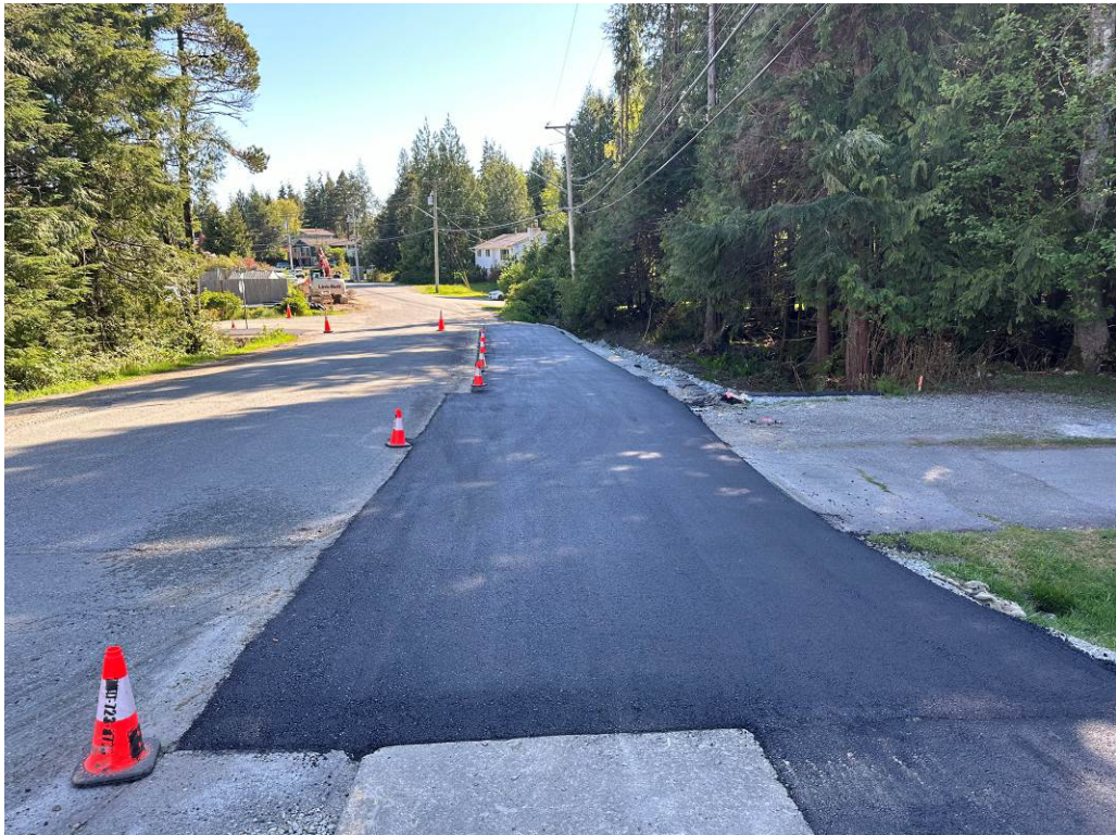
Photo #4 – Bay Steet Pathway – Paving in Progress
