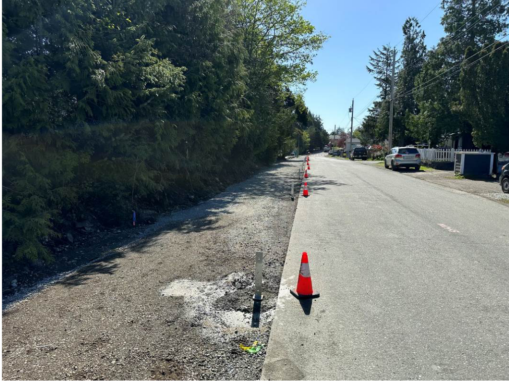
Photo #1 – Larch Road Pathway – Bollard Installation in Progress
