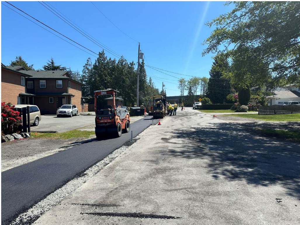
Photo #8 – Larch Road Pathway – Paving in Progress
