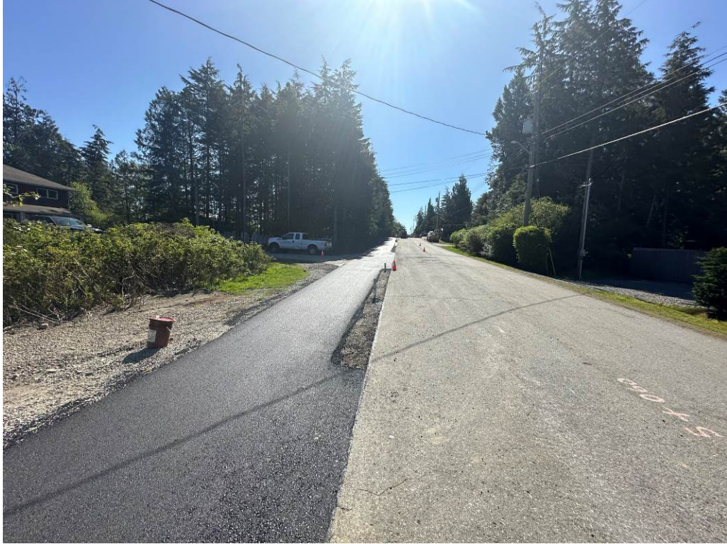
Photo #5 – Larch Road Pathway – Paving in Progress
