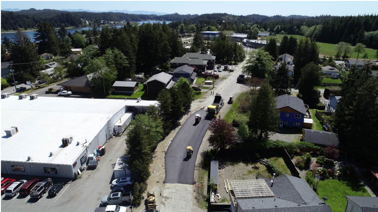
Photo #10 – Larch Road – Paving in Progress
