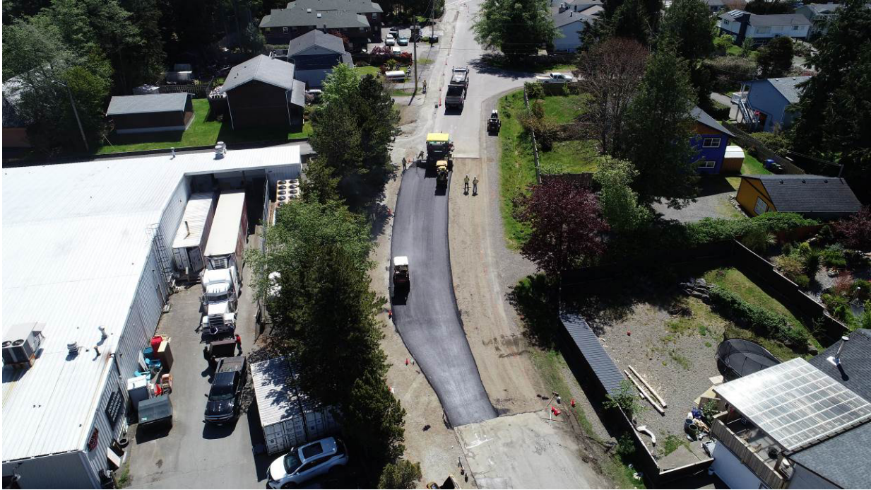
Photo #9 – Larch Road – Paving in Progress
