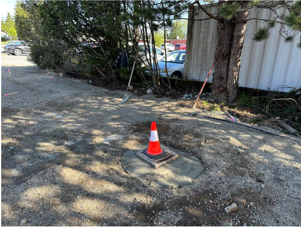
Photo #3 – Catch Basins Adjusted to Finished Grade
