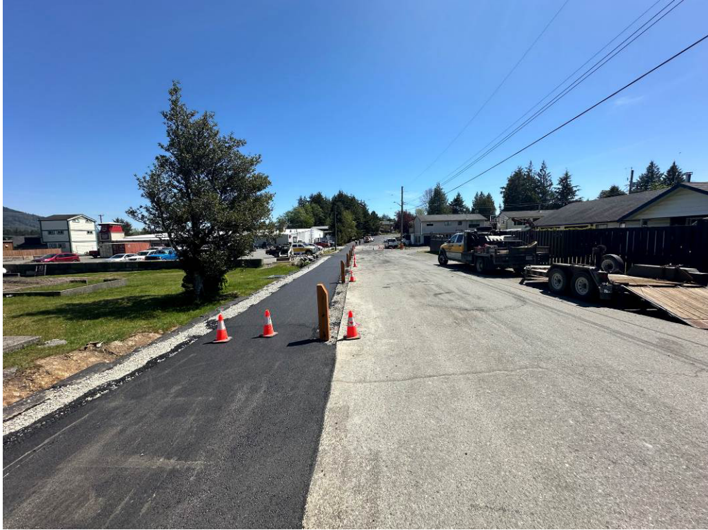
Photo #7 – Larch Road Pathway – Paving in Progress
