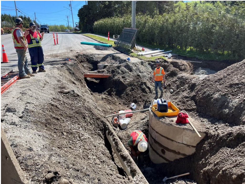
Photo #4 – Catch Basin Installations Ongoing
