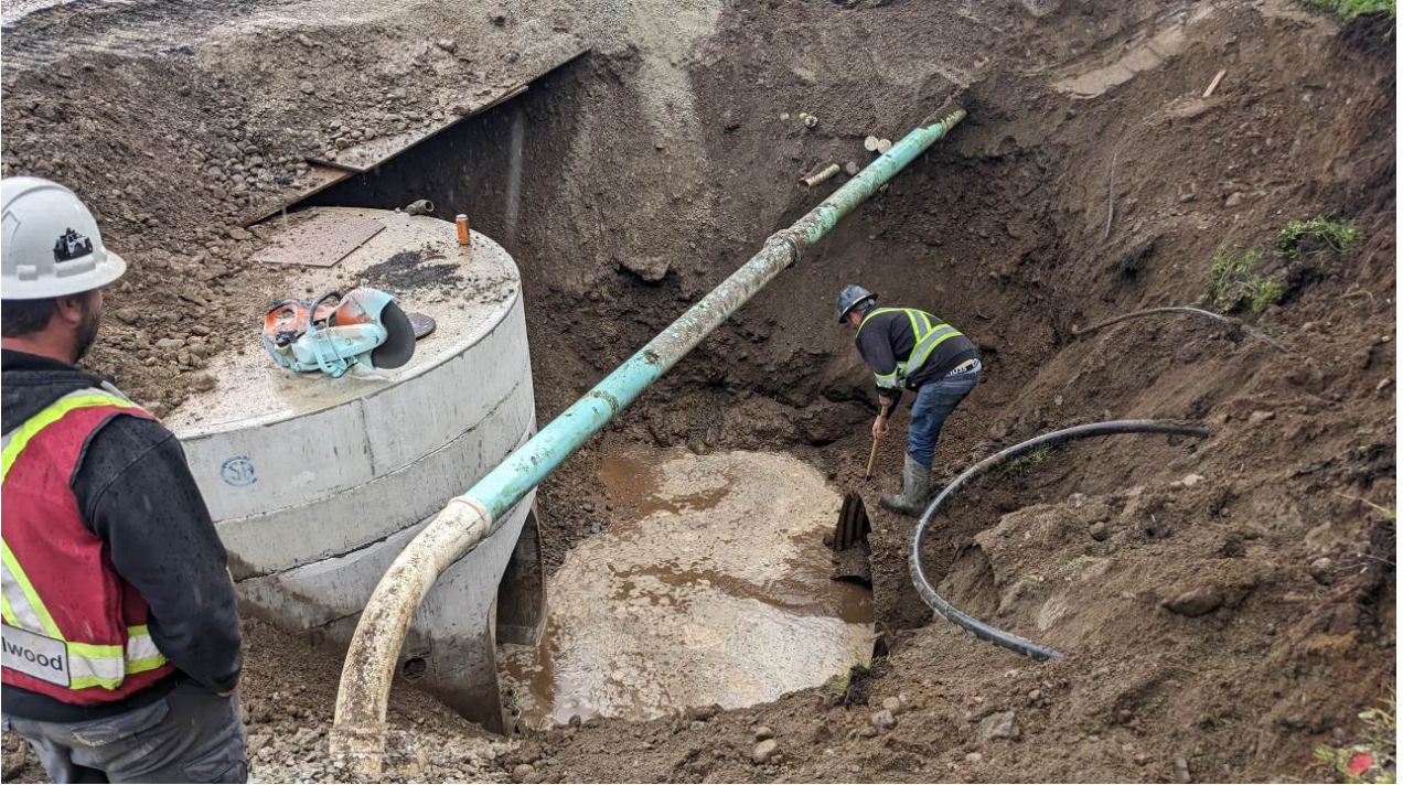
Photo #1 – Connection from DMH #6 to CSP Pipe from Unnamed Stream #4 Completed
