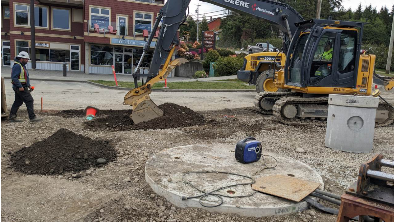
Photo #5 – Catch Basin Installations Ongoing
