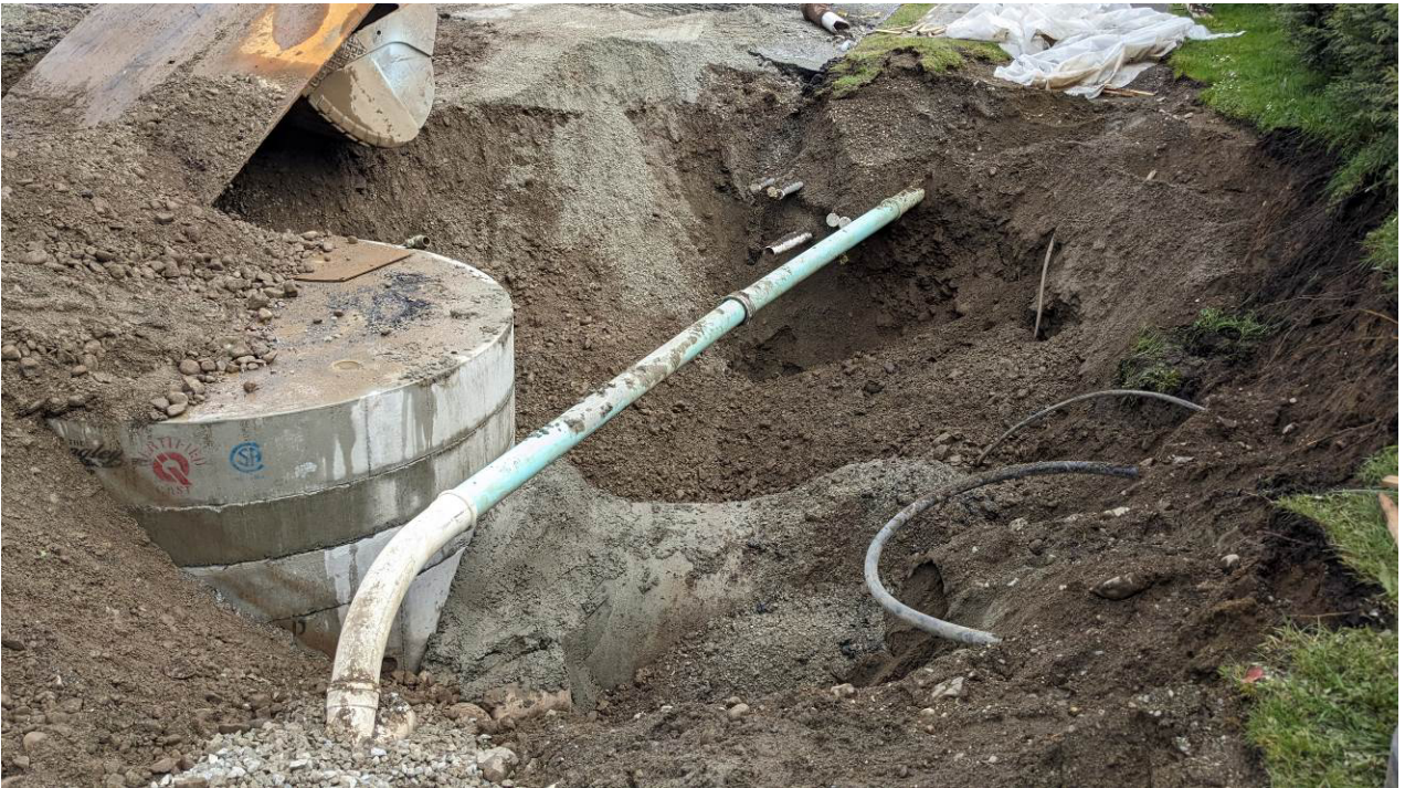
Photo #2 – Connection from DMH #6 to CSP Pipe from Unnamed Stream #4 Completed
