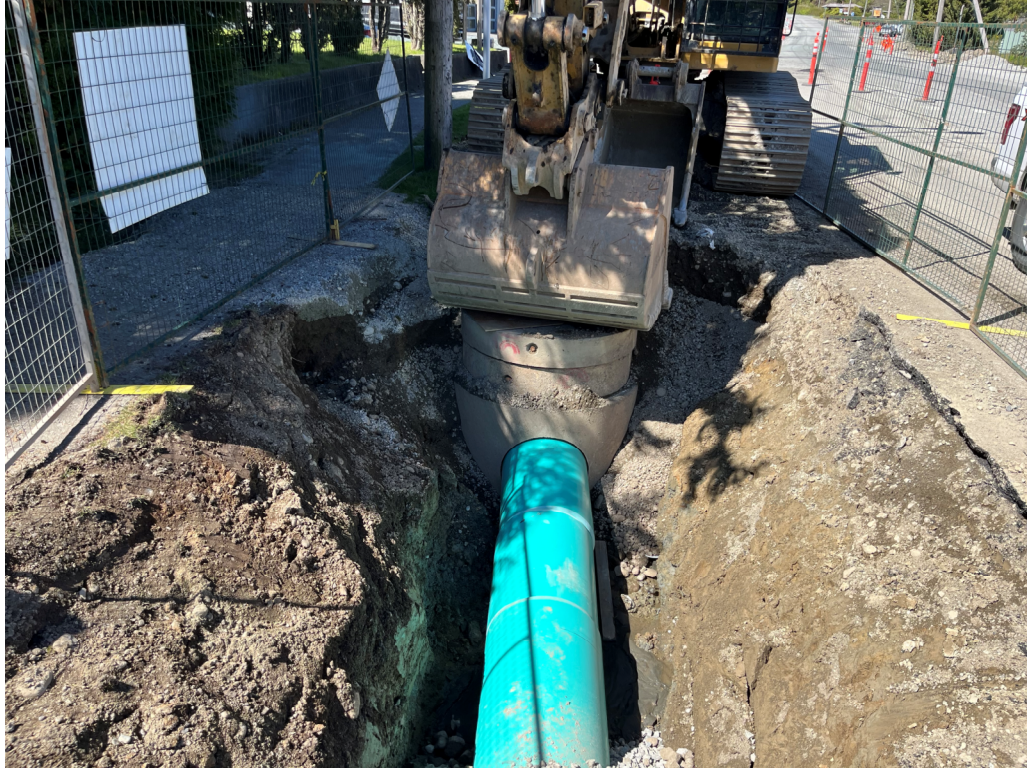
Photo #3 – Storm Pipe Installed from DMH #6 to DMH #5
