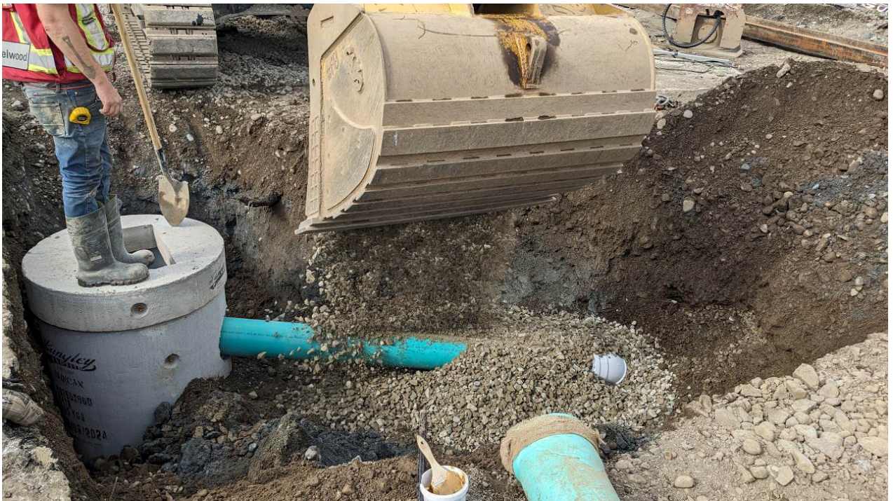
Photo #6 – Catch Basin Installations Ongoing
