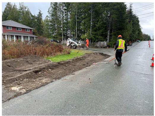
Photo #3 – Larch Road Pathway – Roadway Widening in Progress (5+070)
