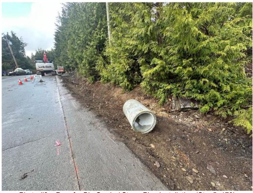
Photo #2 – Prep for Bio-Swale / Storm Pipe Installation (Sta. 5+170)
