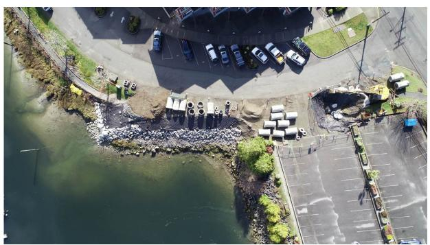
Photo #4 – Erosion occurring at temporary connection between Existing CSP & New Concrete. Hazelwood working on improvements while waiting for manholes to be delivered.
