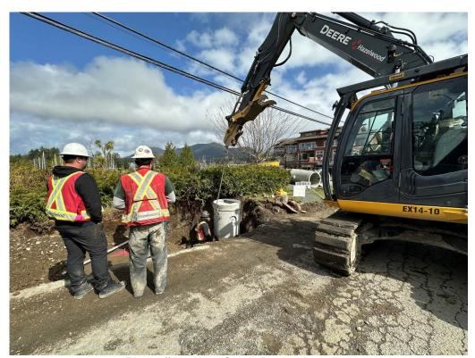
Photo #1 – New Catch Basins Installed
