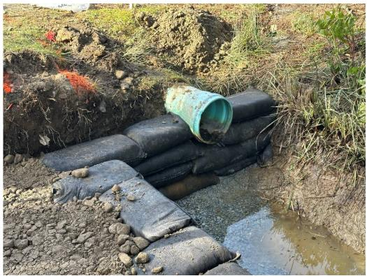
Photo #3 – MSE wall Headwall for Existing Culvert
