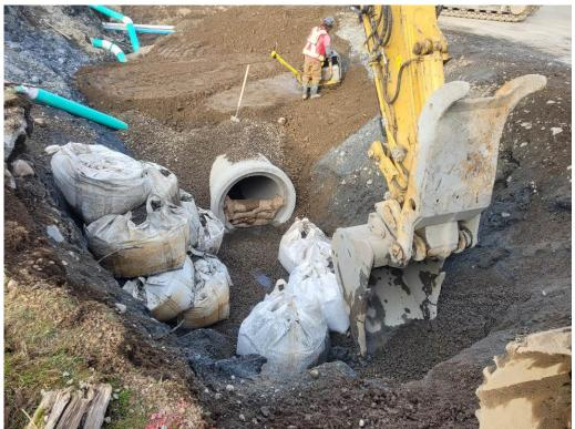
Photo #7 - Temporary Connection Established between New Concrete Pipe & Old CSP
