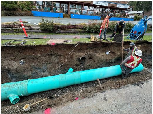
Photo #2 – Peninsula Road Storm System Replacement (DMH #4 towards DMH #3)
