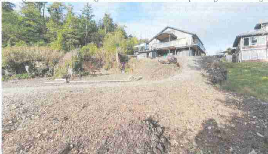
Photo 3. Looking north toward the house. Photos shows spread out soil material, trail, and sloped areas.
