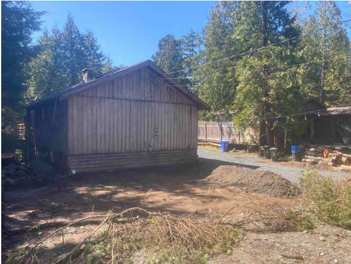
Photo 1. Showing area previously cleared, leveled and compacted for the proposed addition. It is understood no additional clearing is needed for the addition.
