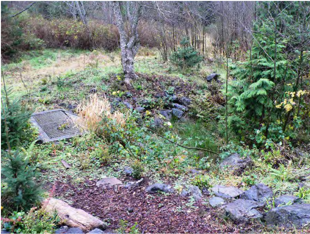
Photograph 1. View from Big Beach access trail to stormwater outlet headwall & grate.
