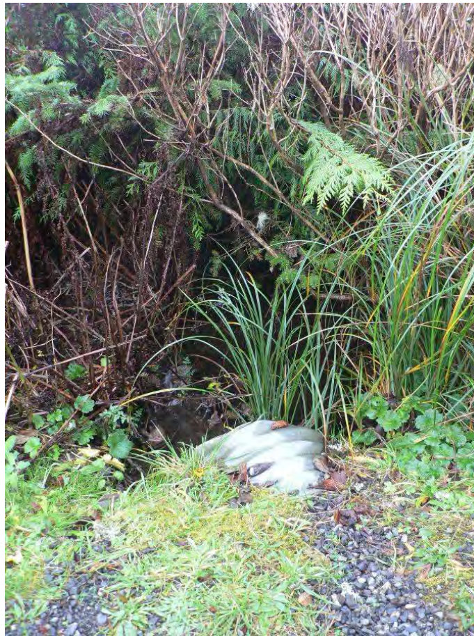
Photograph 4. View of culvert under beach trail.
