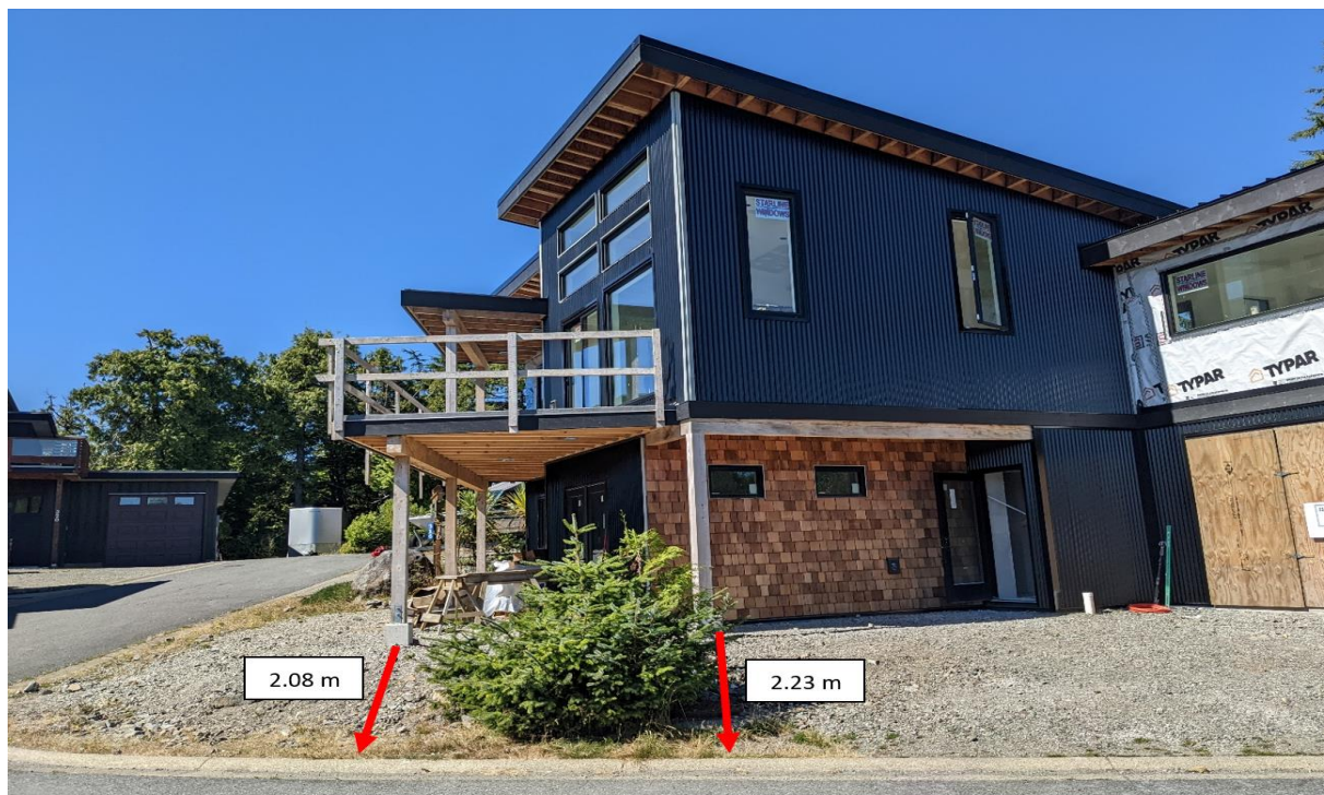
Figure 3 - Photo of post locations
