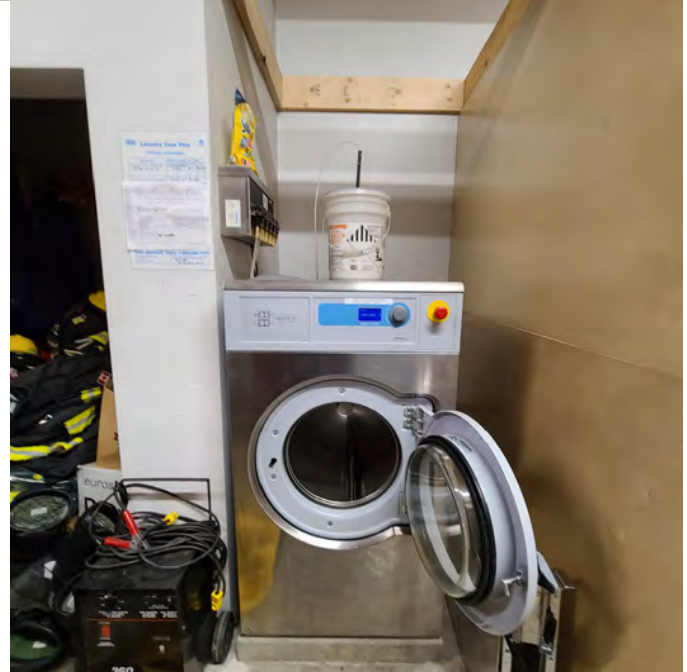
The photo above shows the gear washing machine. No organization or cleaning storage room is available in this area. The workshop storage to the left makes for a non-functional space.
