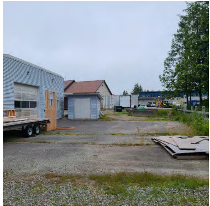
Photo above shows rear yard area. Storage and movement space is limited for trailer storage or other goods. The rear concrete apron has failed. It is assumed that the ground requires structural upgrades to support heavier equipment and training.
