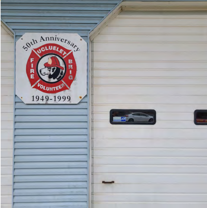
The photo above shows the old Fire Hall branding which is in the process of re-branding. Limited apparatus bay natural lighting or security view toward apron.
