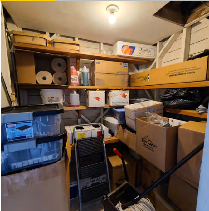
The photo above shows the storage/ janitorial supply room. The room is overstocked and relatively inaccessible due to inadequate shelving and storage space. There is no mop sink for proper cleaning uses.
