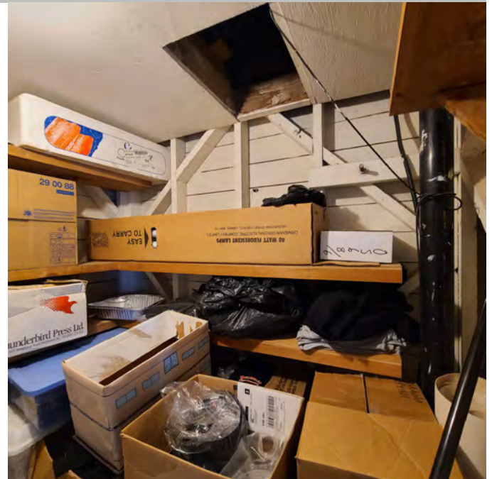
The photo above shows the storage/ janitorial supply room which is accessible in the kitchen area only. The room is unfinished inside with an inaccessible 'attic' access opening in the ceiling.
