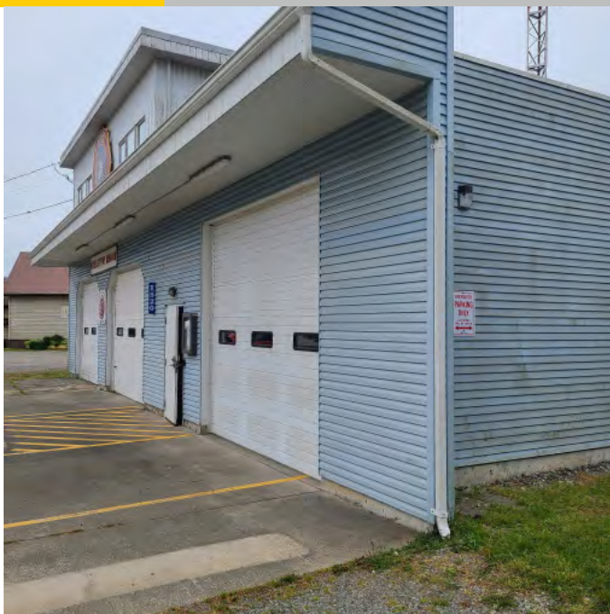
Photo above shows front soffit area/ canopy overhang with surface mounted linear lighting. General lighting appears to be inadequate for an emergency facility. Downspouts appear to be undersized residential style. OH doors show signs of wear and weathering.
