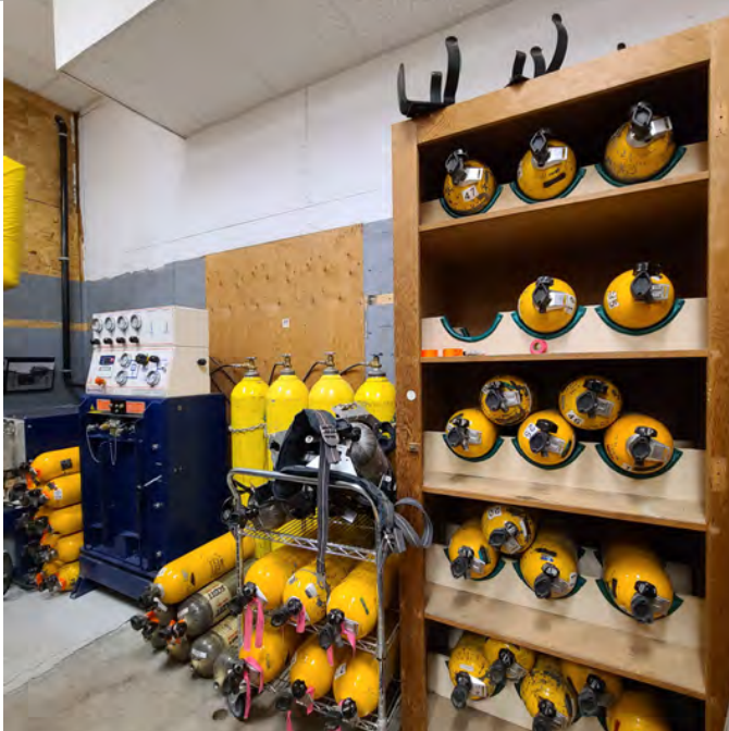
The photo above further highlights the issues noted in the photo to the left. SCBA and compressors require a dedicated 'clean room' for proper separation from apparatus bays and intake of fresh air. Clean work area is needed for storage and maintenance of equipment.
