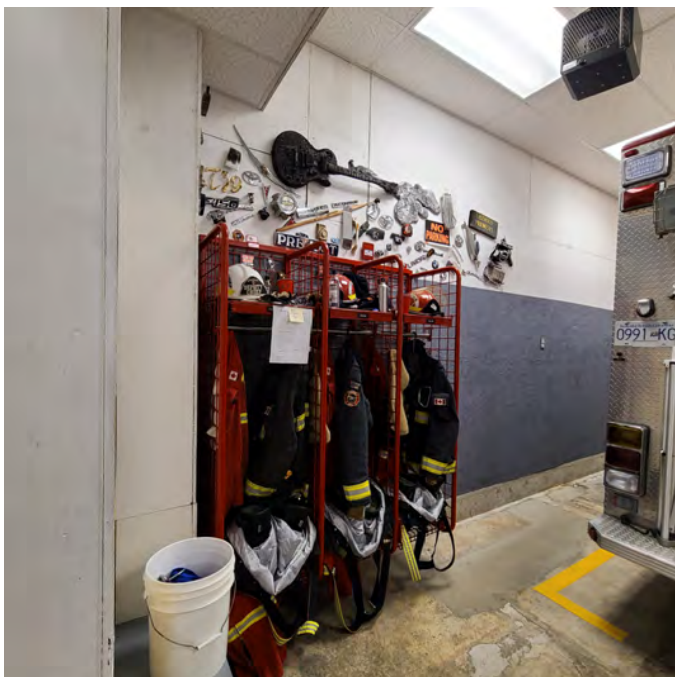
The photo above shows a 3-tier ready rack system hung at the back of the main apparatus bays. There is not enough room for the gear to be hung all in the same room. The gear layout is scattered and inefficient. A proper sized gear room is required.
