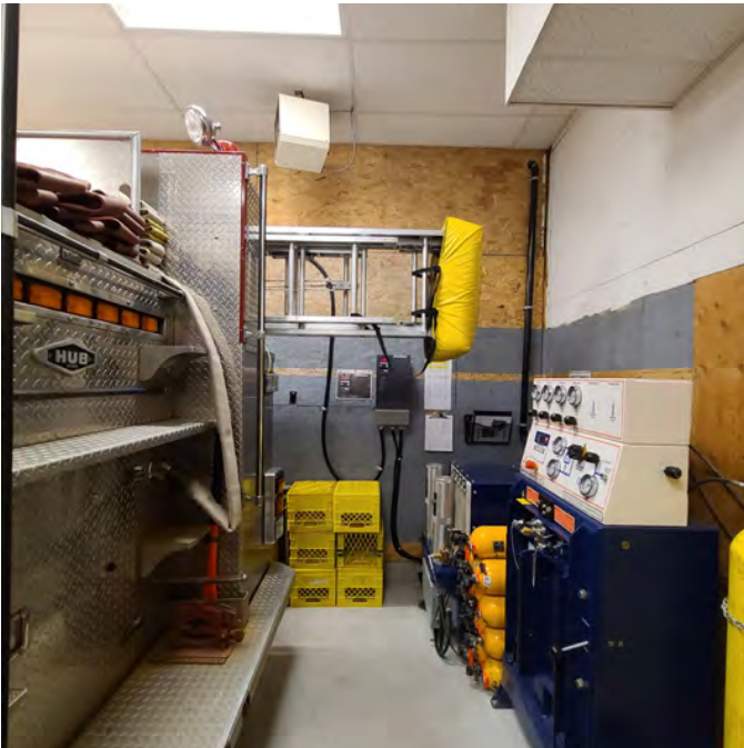
The photo above shows a ladder protruding from the back of the fire truck which poses a safety hazard and movement limitations. The SCBA and compressor should be relocated and items should not be stored in this area.
