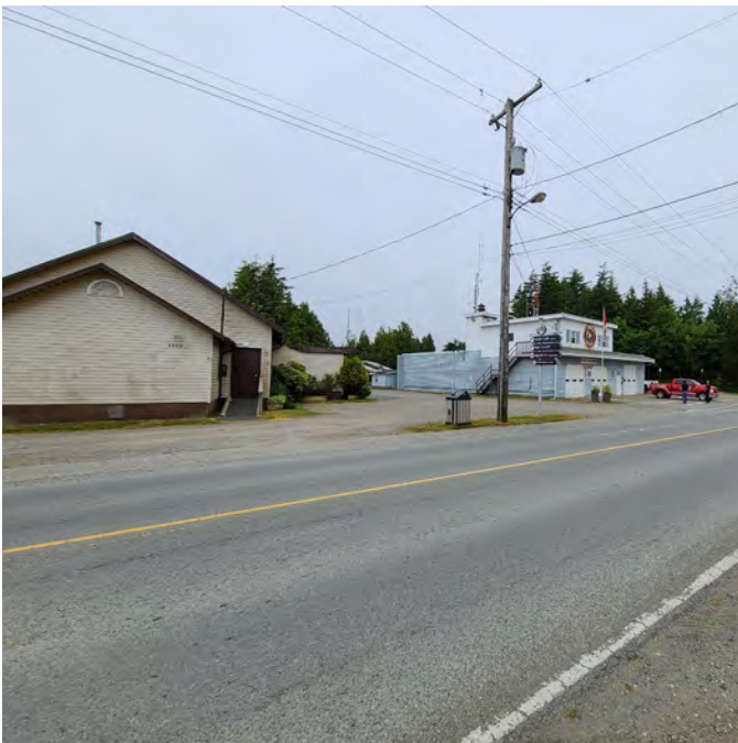
The photo above shows an overall view of the UAC and Fire Hall sites. Both are on generally flat, level ground which would be ideal for building on. These sites are outside the District Tsunami Hazard zone. It would be desirable to run hydro underground from the pole.
