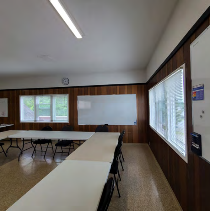
The photo above shows a further look at the training area. The room has good natural lighting. The windows need to be replaced with new. The lighting should be upgraded.
