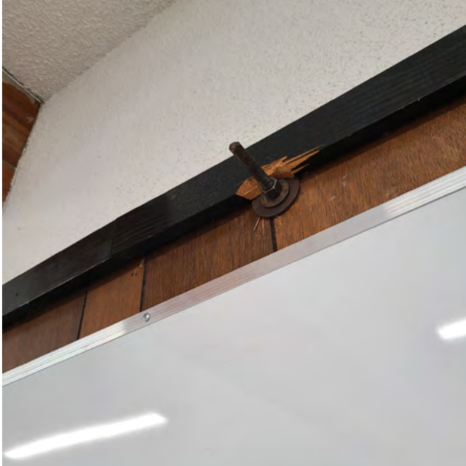
The photo above shows a through-wall bolt connection (purpose unknown).
