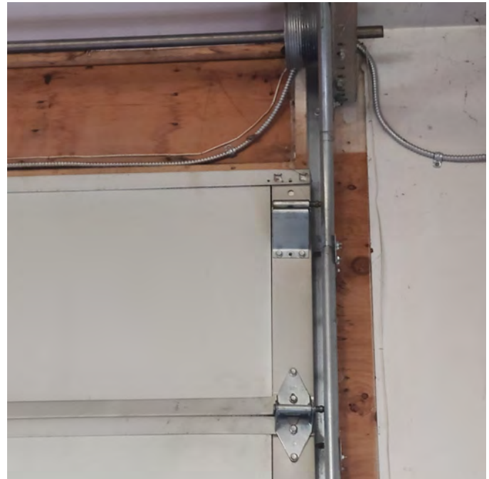
The photo above shows the bay addition overhead door mounting.
