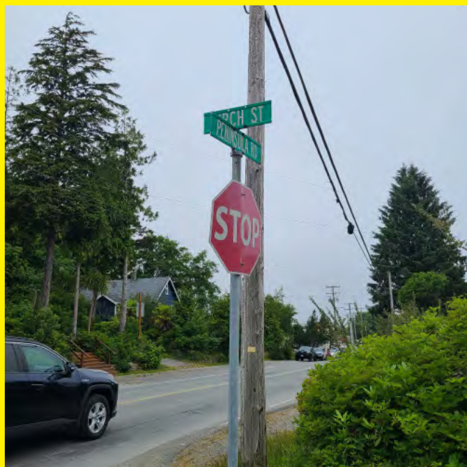
Photo above shows Peninsula Rd./ Birch St. intersection controlled only by a 'stop' sign. Fire Hall access and egress should be controlled by flashing traffic lights for traffic safety due to lane blockages (quick departures/ slow returns backing in off road)
