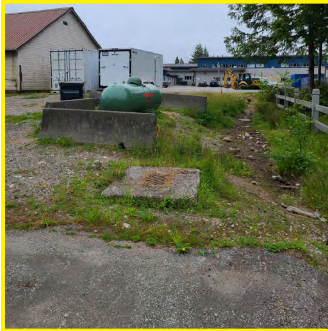
The photo above shows potential site hazard areas. While the propane tank is protected, the security level is low. This area shows much site deterioration and blocks much movement and training area. This needs to be relocated and site repairs are needed.
