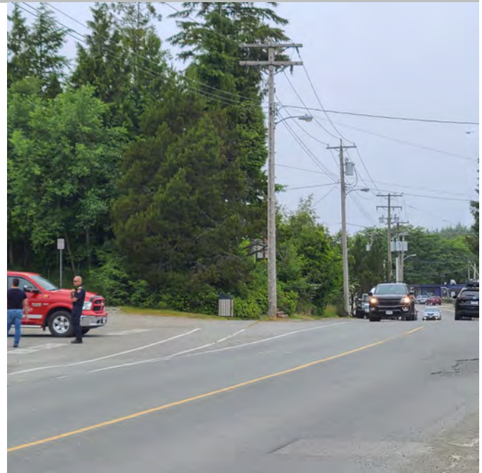
The photo above shows northbound and southbound traffic lanes along Peninsula Rd. in front of the Fire Hall. Traffic levels appear consistent along this main town thoroughfare. Roadway lines should be upgraded to ensure Fire Hall apron is not blocked by traffic stops.
