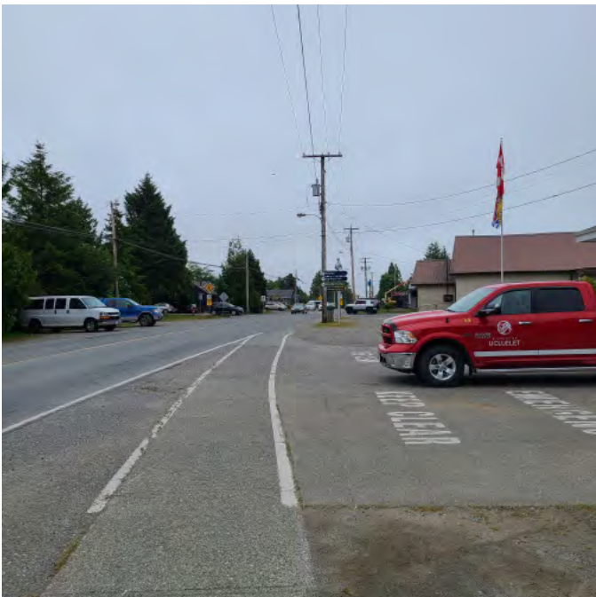
Photo above shows site frontage along Peninsula Rd. (South) There are no flashing lights to control traffic when entering or exiting the Fire Hall. Walking and traffic lanes are shown above with no proper apron delineation. Site grading changes are also required.
