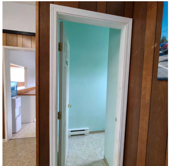
The photo above shows one washroom with electric baseboard heating.
