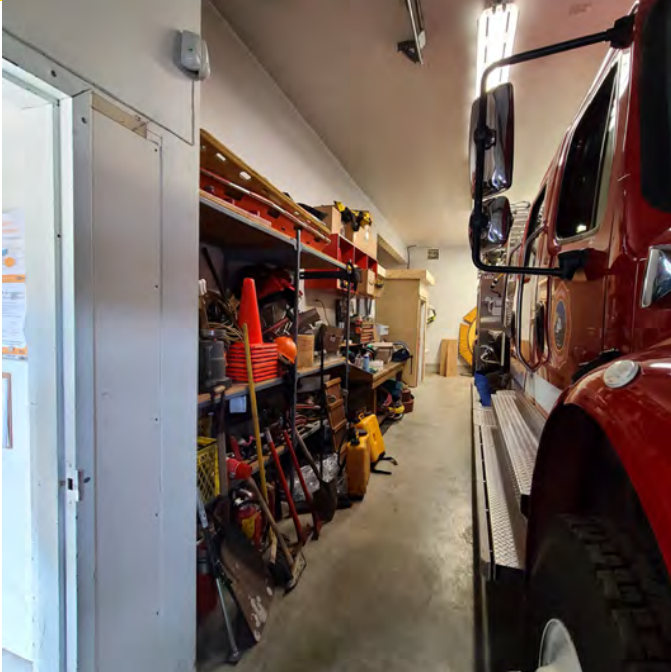
The photo above shows a look at the 'work shop' area located in the 3rd apparatus bay (left side of bay). There is not enough room for proper tool, equipment, and fuel storage.
