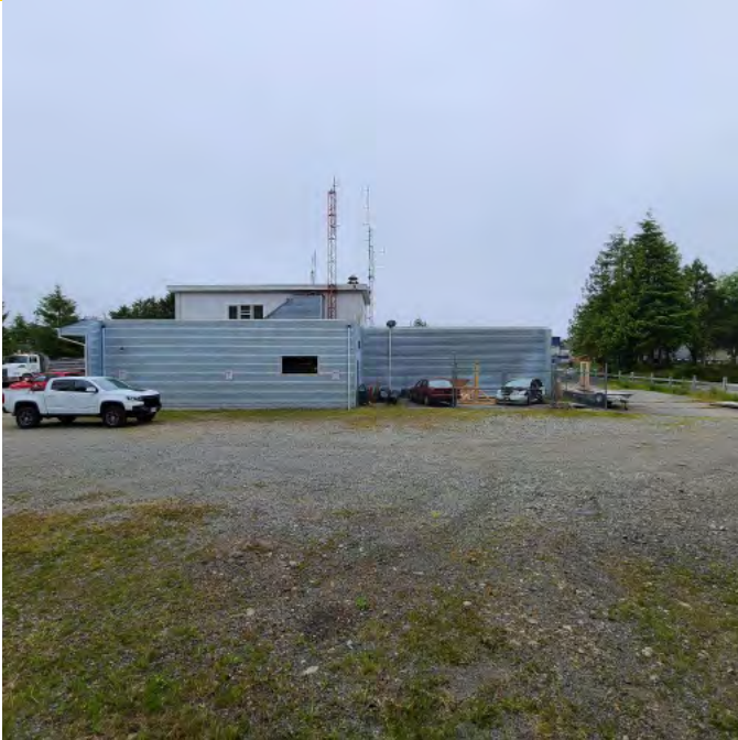
Photo above shows the Fire Hall side (North) elevation and training storage area. The general site conditions are degrading and require upgrade and maintenance.
