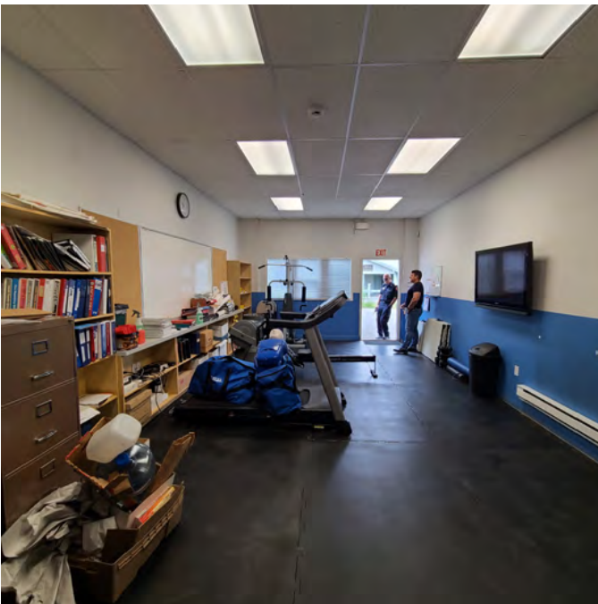
The photo above shows an overall look at the main floor admin. area and gym. Baseboard heating is observed, painted drywall and acoustic ceiling tile finishes.
