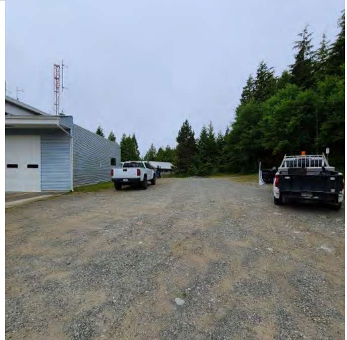
Photo above shows secondary informal gravel apron access to the Fire Hall property from Peninsula Rd. This area of the property is used for parking and training purposes. This area is too small for required uses. Too small for proper truck turning, training, and parking.
