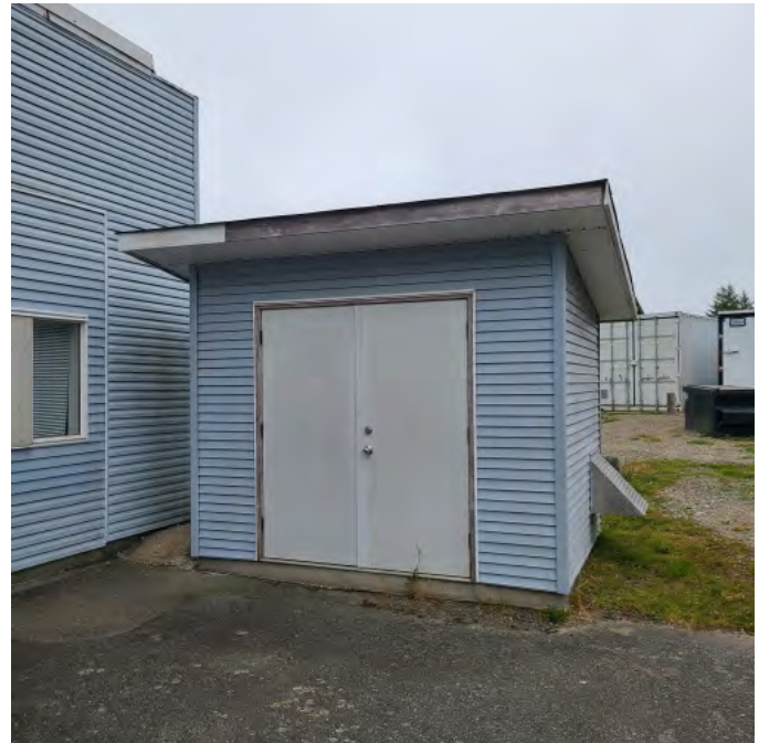
The photo above shows an added exterior shed. The shed is showing similar signs of wear and degradation. An upgraded Fire Hall would cover this footprint area.
