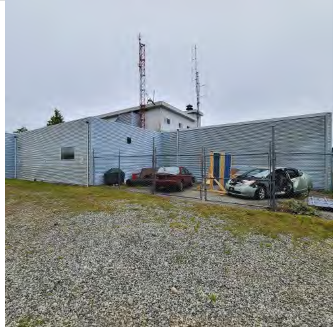
Photo above shows exterior training storage area for vehicles and other equipment or practice materials. Storage space is limited and has low level security. Exterior lighting is limited and not sufficient for night training activities.
