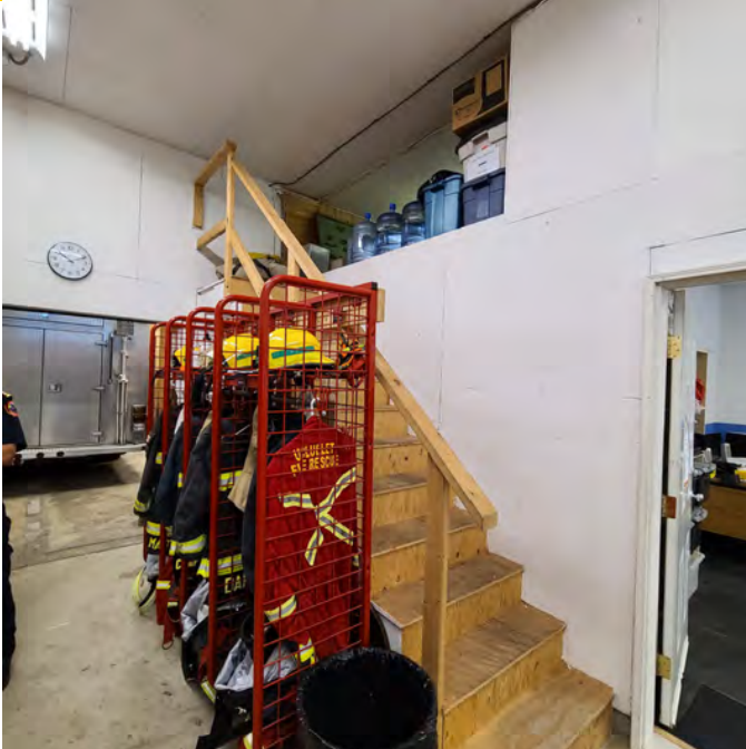
The photo above shows the access stairs to the storage mezzanine and the door entering the office, gym, and radio rooms to the right. The storage space is not safely accessible.
