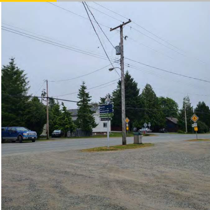
The photo above shows the overhead hydro lines feeding the Fire Hall. There is no post protection to prevent pole damage and possible power outages. Some traffic control signage is noted between the Fire Hall and USS. Neighbouring properties seen in photo.
