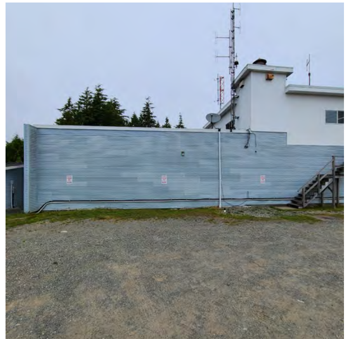
The photo above shows an exterior view of the lower level administrative building components. No parking is available along this facade. The flat roof drains through scuppers and downspouts as shown in the photo above.
