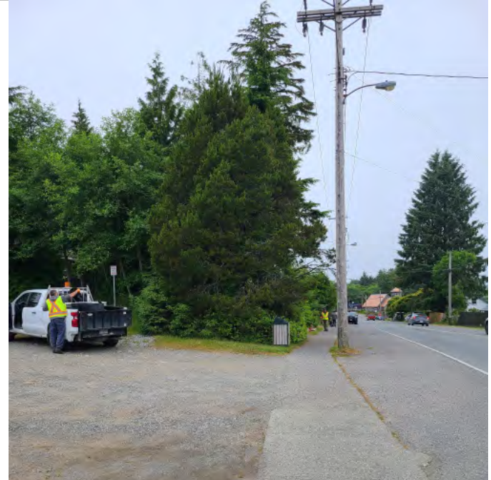
Photo above shows hydro lines along Peninsula Rd. District workers also using Fire Hall lot for temporary purposes.
