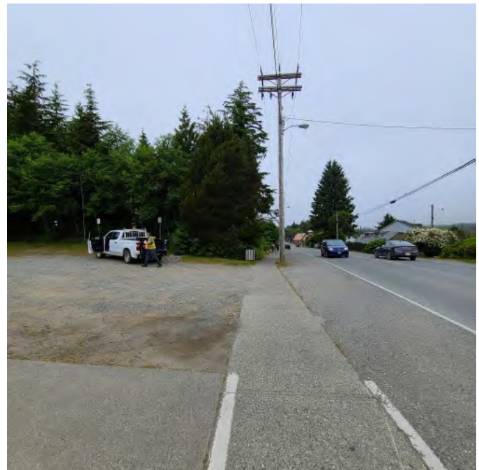
Photo above shows site frontage along Peninsula Rd. (North). Gravel yard area spills debris onto roadway. Trucks block traffic when entering and exiting site. No apron delineation is present. Tree line shown in photo approximately marks lot line.
