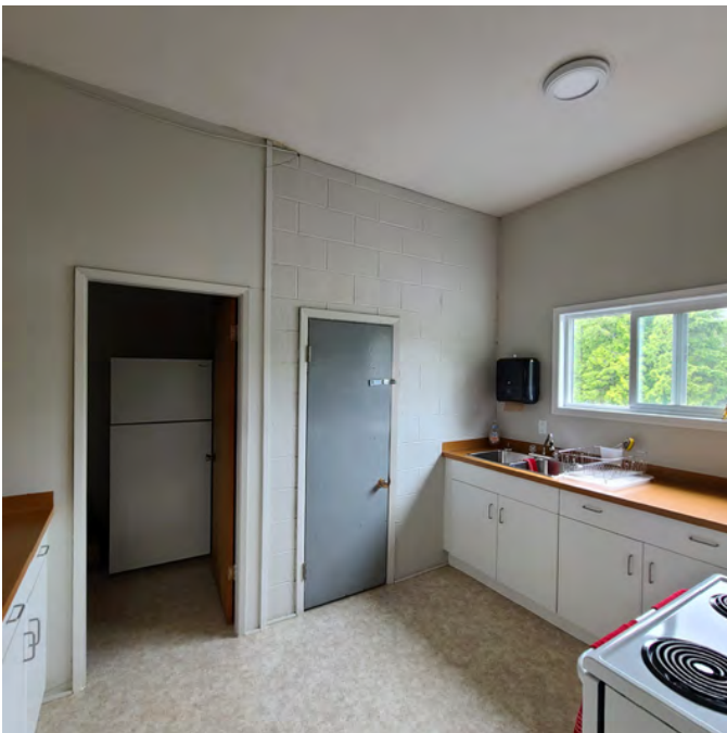
The photo above shows a view of the general kitchen layout. There is no room for the fridge to be placed within the required space.
