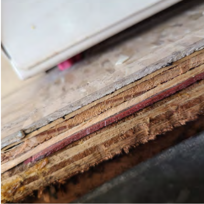
The photo above shows multiple flooring layers.
