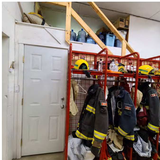
The photo above shows access to a small storage area under the staircase with a small storage mezzanine above and a 4-tier ready racking system to the right.
