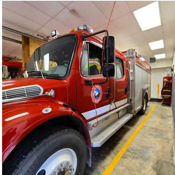
The photo above shows one of the Fire Hall apparatus bays. Walking room is generally clear but is very tight according to industry standards. The ceiling finish height is low. Lighting is just sufficient. The concrete floor is worn and stained.
