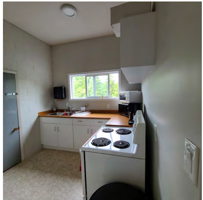
The photo above shows an overall outdated kitchen that needs redesign. More counter space and prep. area is required.
