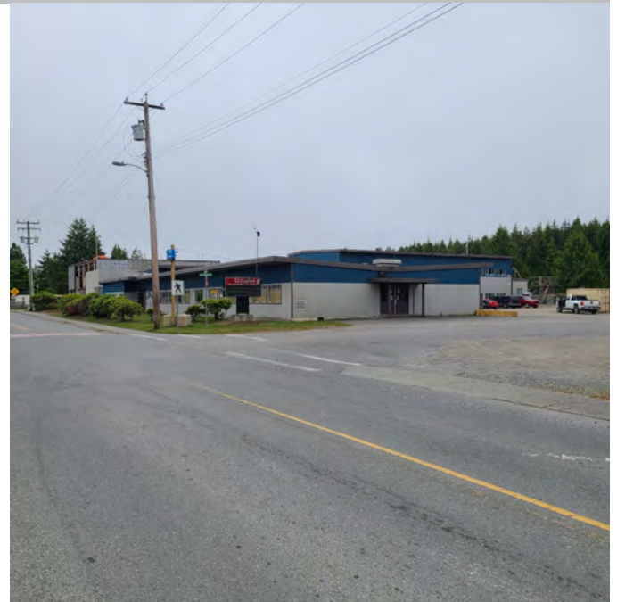
The photo above shows an overall view of USS with the addition and renovation work seen in the background. It is assumed that the entire school facility will be seismically safe at the end of the project whereas the Fire Hall across the street is not.
