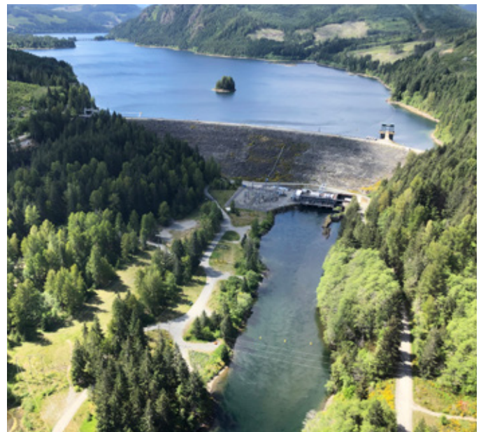
Strathcona Dam, one of the dams in the Campbell River system, is the largest dam on Vancouver Island.
