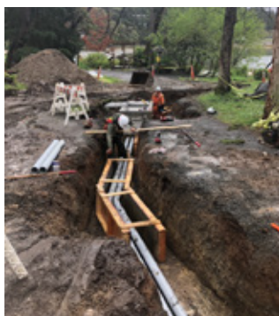
Crews installing conduit on Protection Island.
