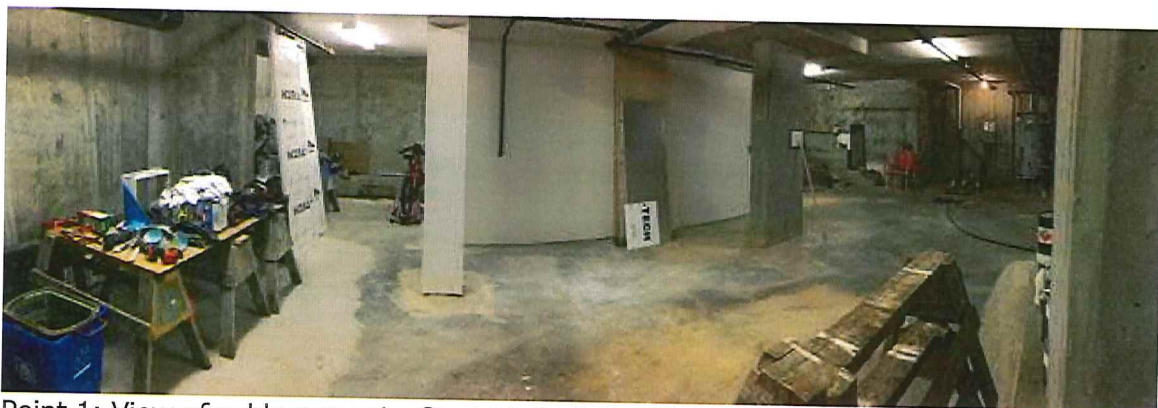
Point 1: View of subbasement - Strata Lots One and Two
