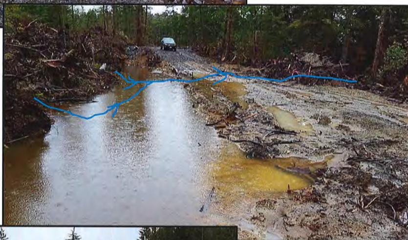
Photo 8: Impacted drainage. Engineer to complete Stormwater management plan for site.
