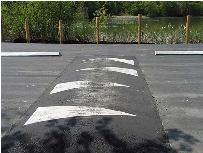
Figure 3: Asphalt Speed Hump
