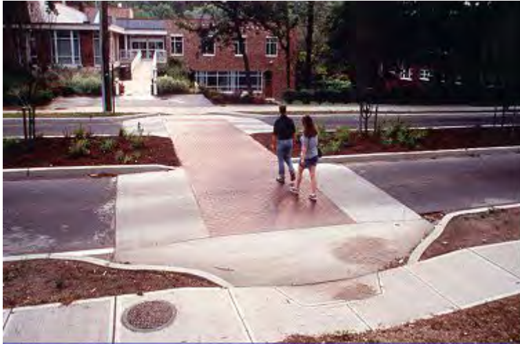
Figure 2: Raised Concrete Crosswalk
