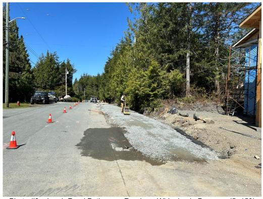
Photo #2 – Larch Road Pathway – Roadway Widening in Progress (5+150)
