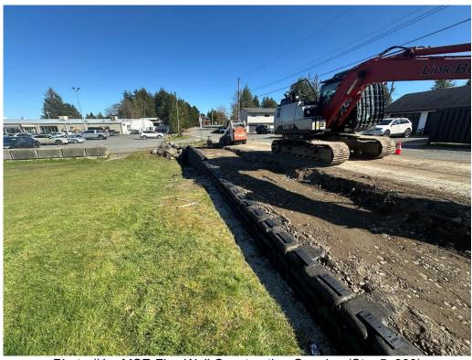
Photo #4 – MSE-Flex Wall Construction Ongoing (Sta. 5+300)
